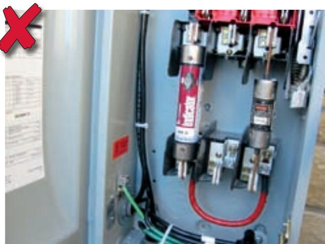
Improper enclosure grounding: wrong device, wrong location.
