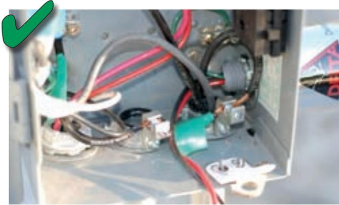
Bonding bushings on 500 VDC conduits.
