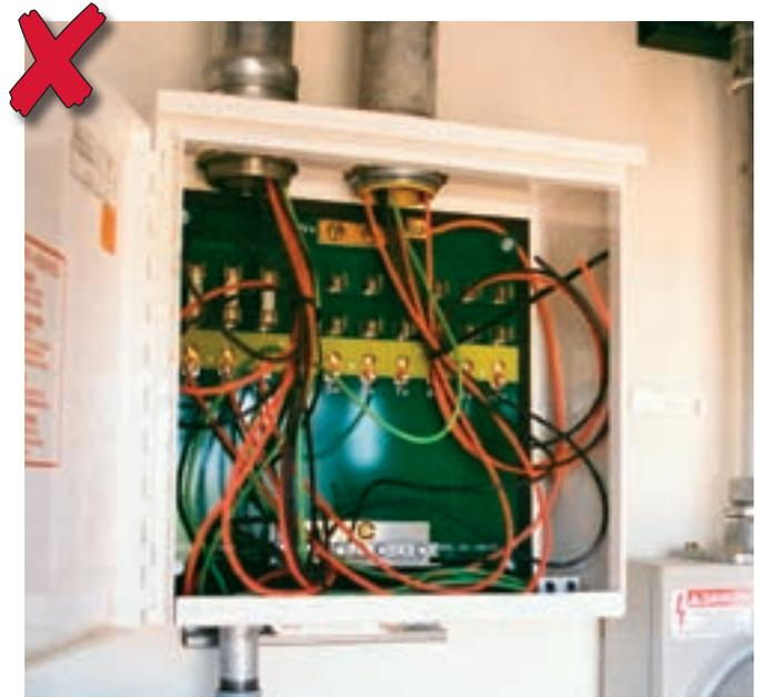
**Grounded PV source circuits, but no white conductors.**
