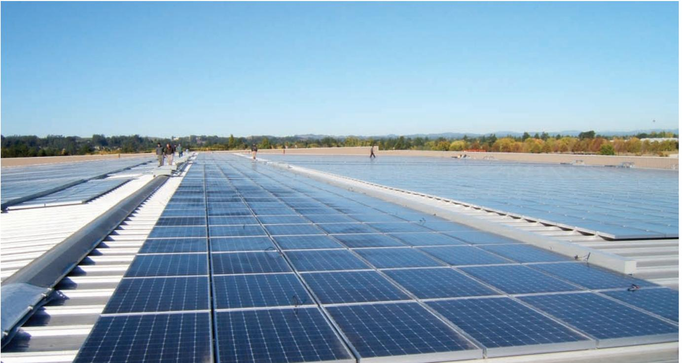
**PV modules and racks must all be properly grounded.**
