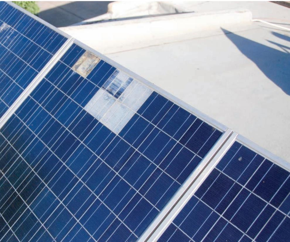
**PV modules do occasionally fail and may create hazardous fault conditions in poorly grounded arrays.**
