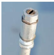
**A cord grip keeps water, critters, and detritus out of a raceway, while allowing the cable to pass through.**
