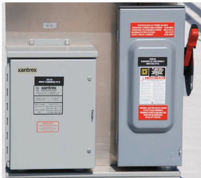
**For large systems with several series strings, a disconnect at the output of every combiner eases servicing the recombiner or inverter fuses.**
