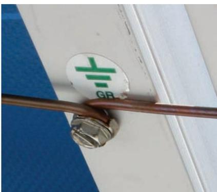
**Although this copper ground appears installed per the module's instruction manual, the copper is touching the aluminum frame which will corrode the aluminum and destroy the electrical contact.**
