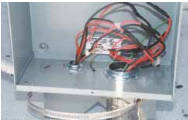
Not to code: improper color coding.
