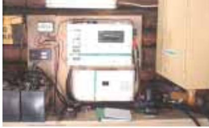
Not to code: DC250 mounted horizontally.
