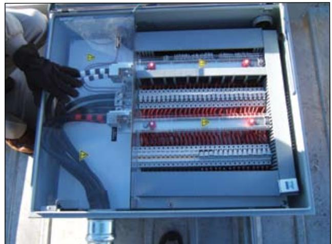
**Photo 3. DC combiner boxes with fuses operating up to 600 volts.**
