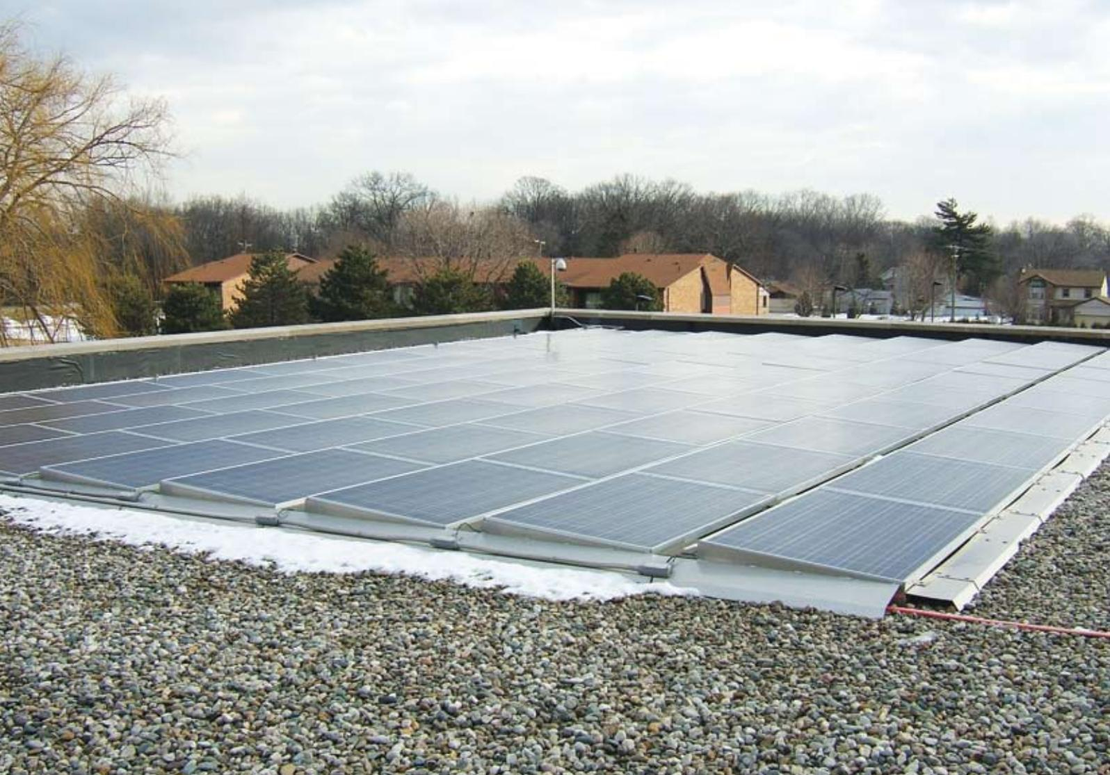
Photo 1. Cold weather increases module open-circuit voltage.
