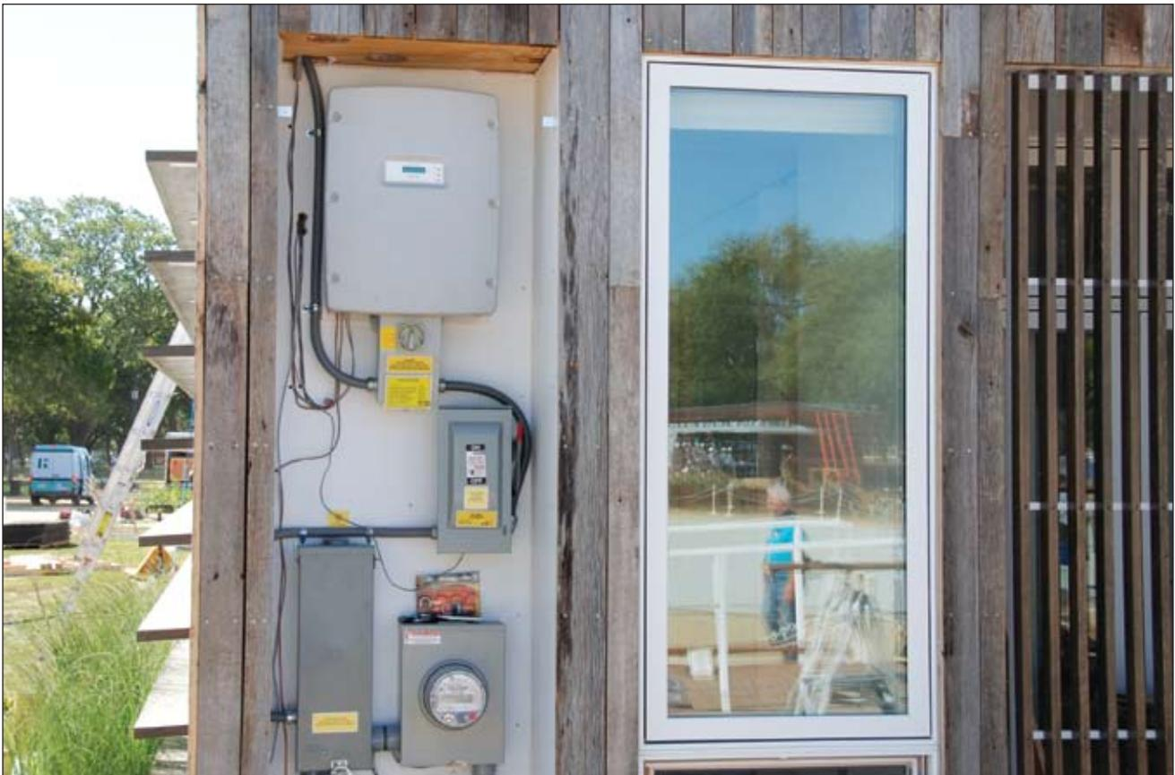
**Photo 4. PV ac disconnect above closed service disconnect**
