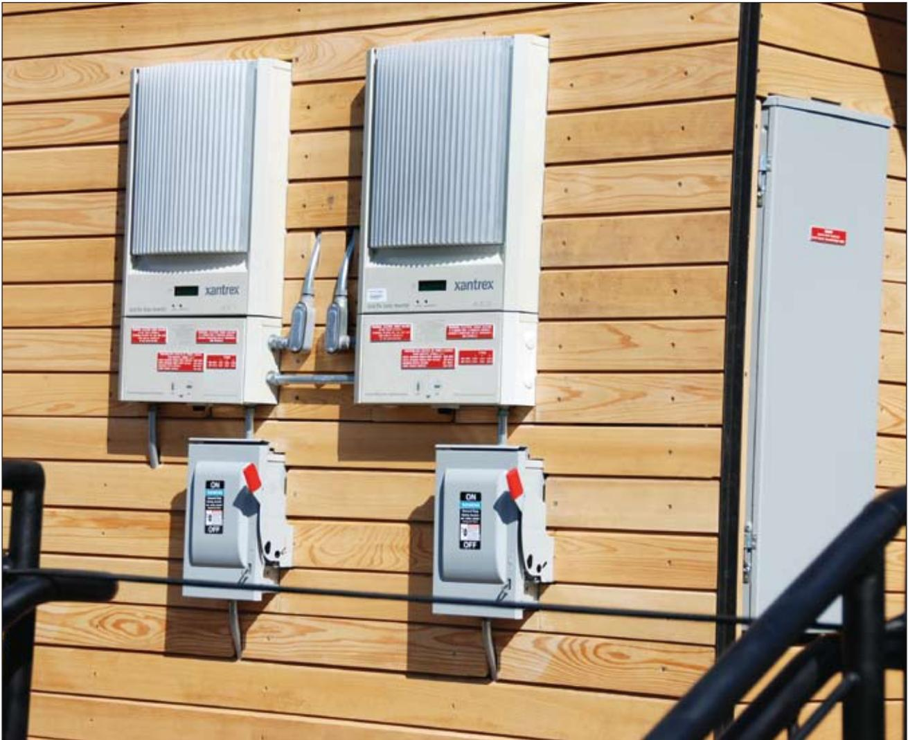
**Photo 2. Utility-required ac disconnects. Could have been combined into one.**
