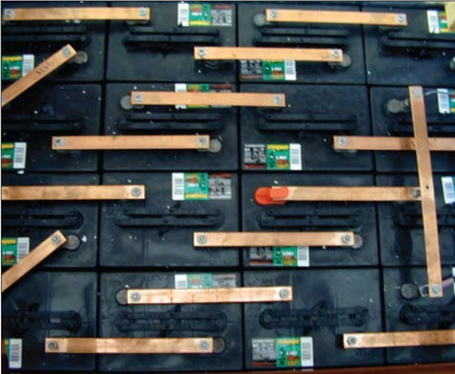
Photo 4. Copper busbars are used instead of cables.
