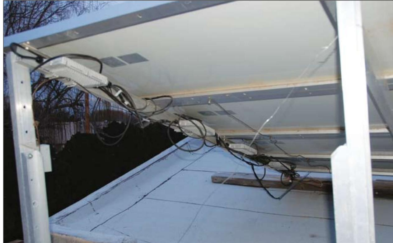
Photo 4. Microinverters — disconnects required?
