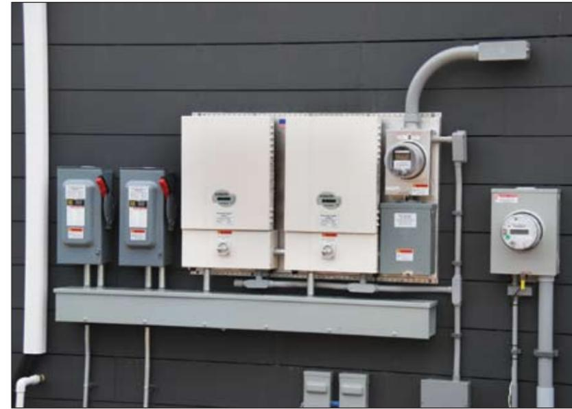
Photo 3. Inverters with internal AC and DC disconnects plus external disconnects
