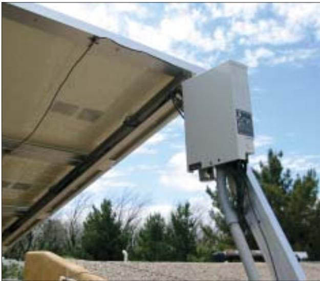
**Photo 5. Combining box wiring**
