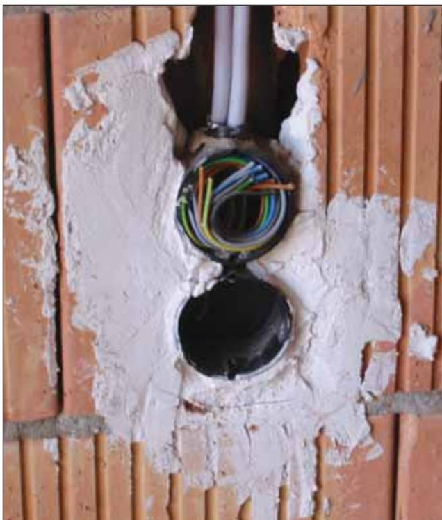
**Photo 4.** Fine stranded cables used for residential wiring
