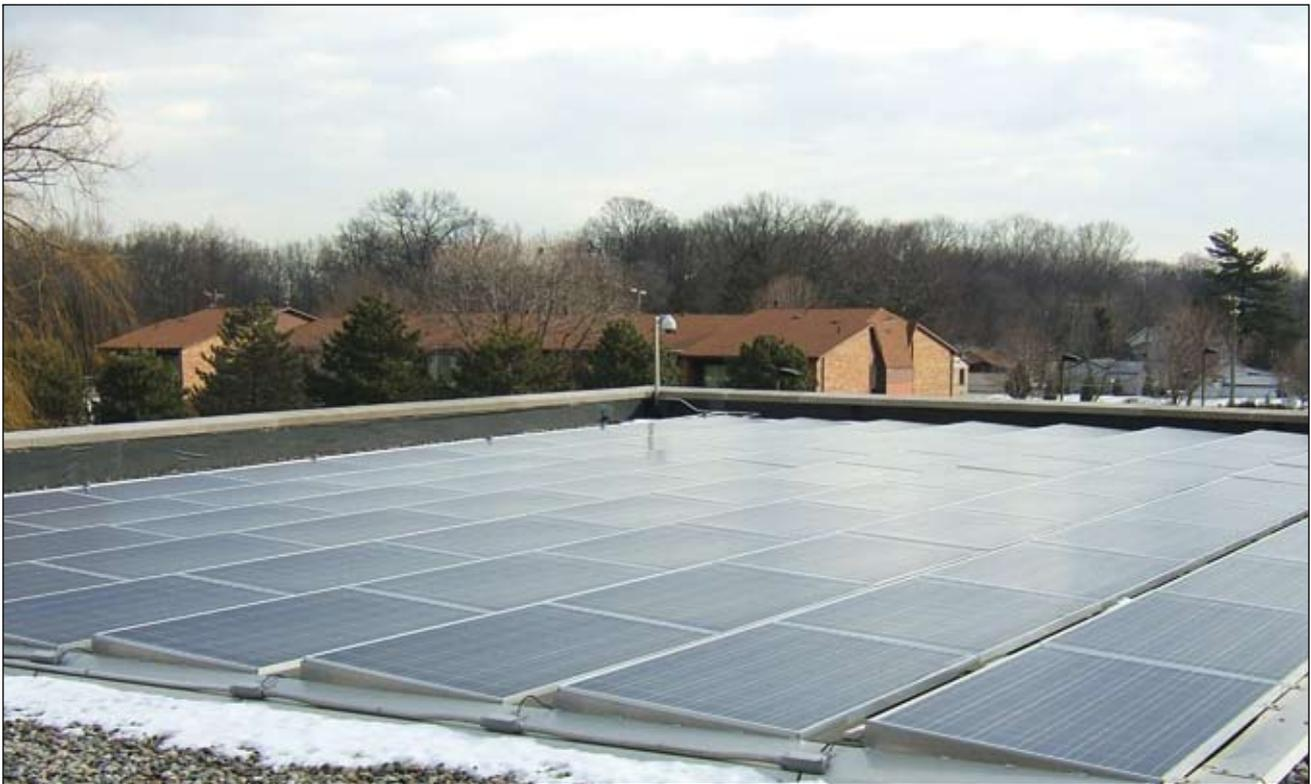
**Photo 3. Cold weather increases module voltages and sunlight helps too.**
