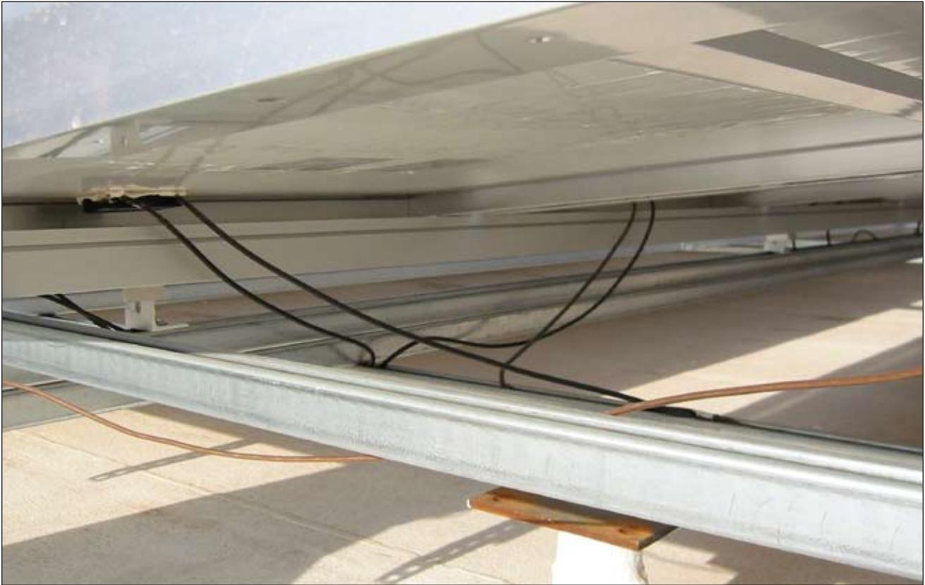
**Photo 2. Improperly secured conductors can abrade and fault.**
