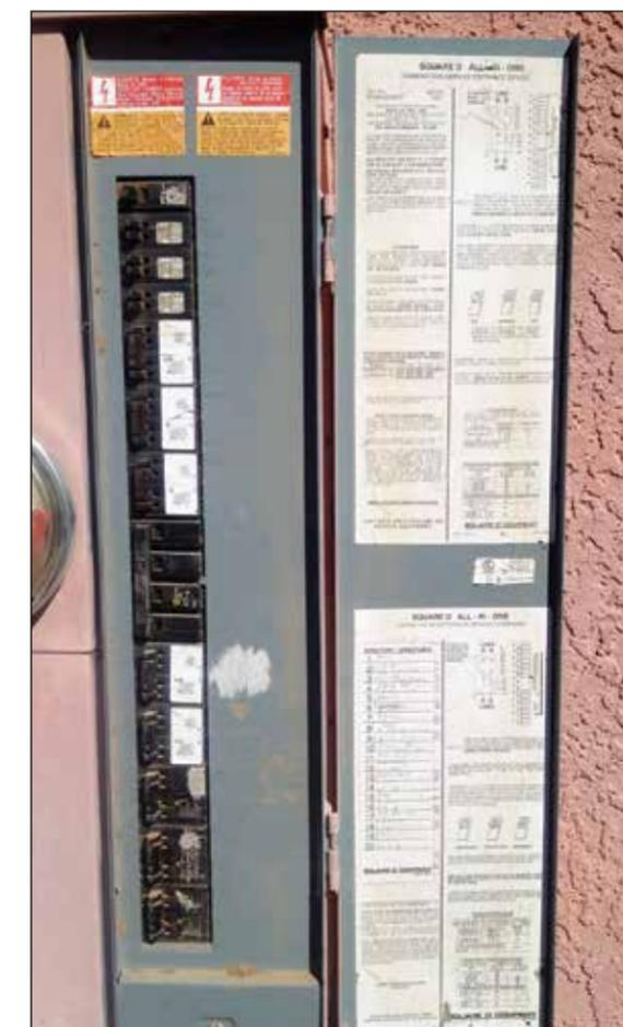
Photo 1. Center-fed Panelboard Courtesy SunSpot Solar
