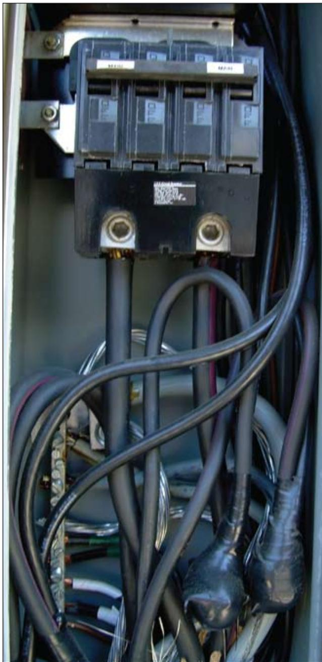
**Photo 3. Load-side connection on output main breaker. Conductors to PV disconnect/overcurrent protection should be as large as the main output conductors.**
