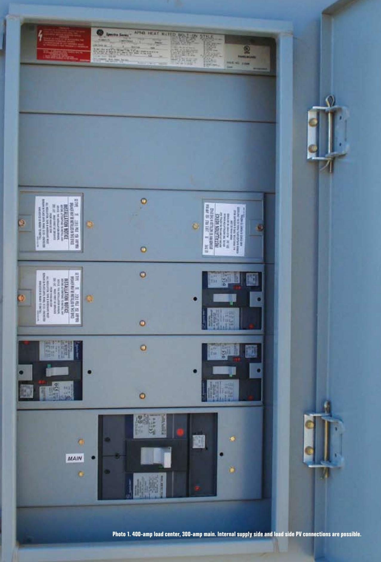
Photo 1. 400-amp load center, 300-amp main. Internal supply side and load side PV connections are possible.
