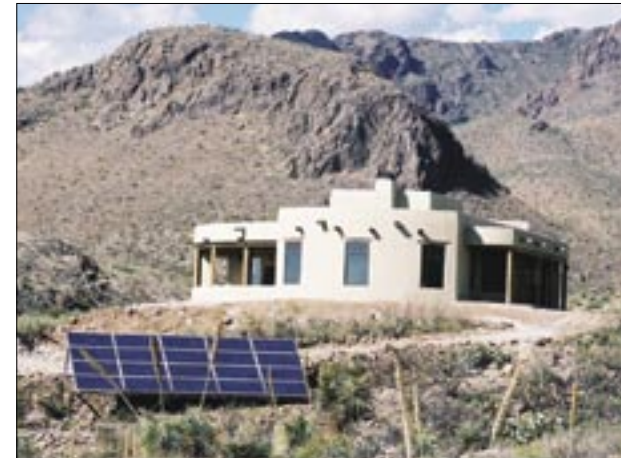
Photo 5. Off-grid home with 3.6 kW PV array
