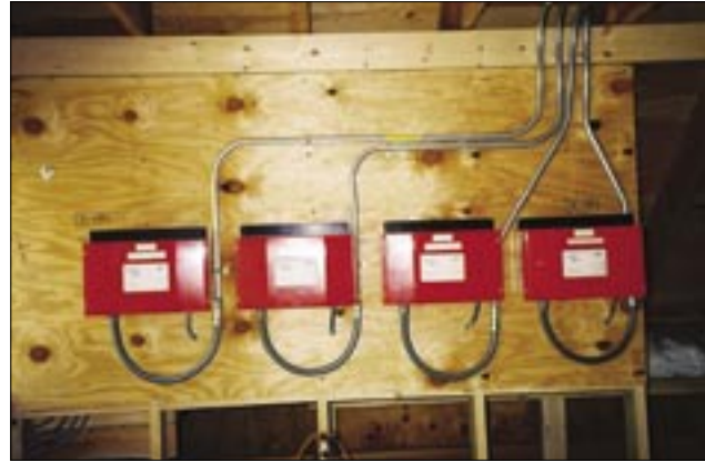
Photo 7. Four 2.5 kW inverters used on a 10 kW utility-interactive residential PV system.
