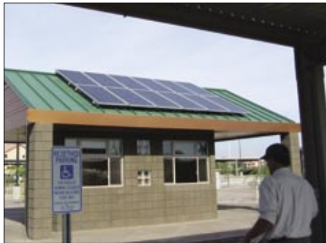
Photo 4. A view from the ground of the smaller 2 kW PV system
