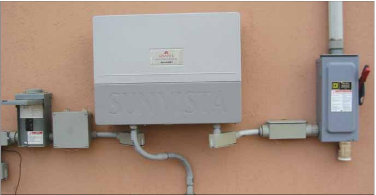
**Photo 4. Inverter with external ac and dc disconnects**
