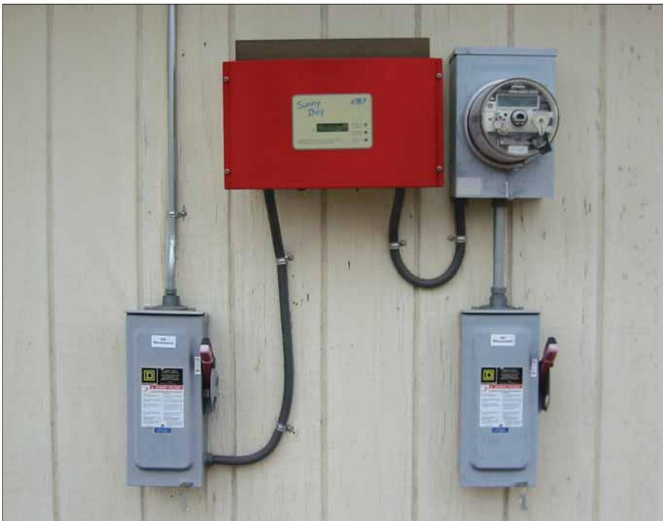
**Photo 5. Inverter ac disconnect combined with the utility disconnect to the right of the inverter**
