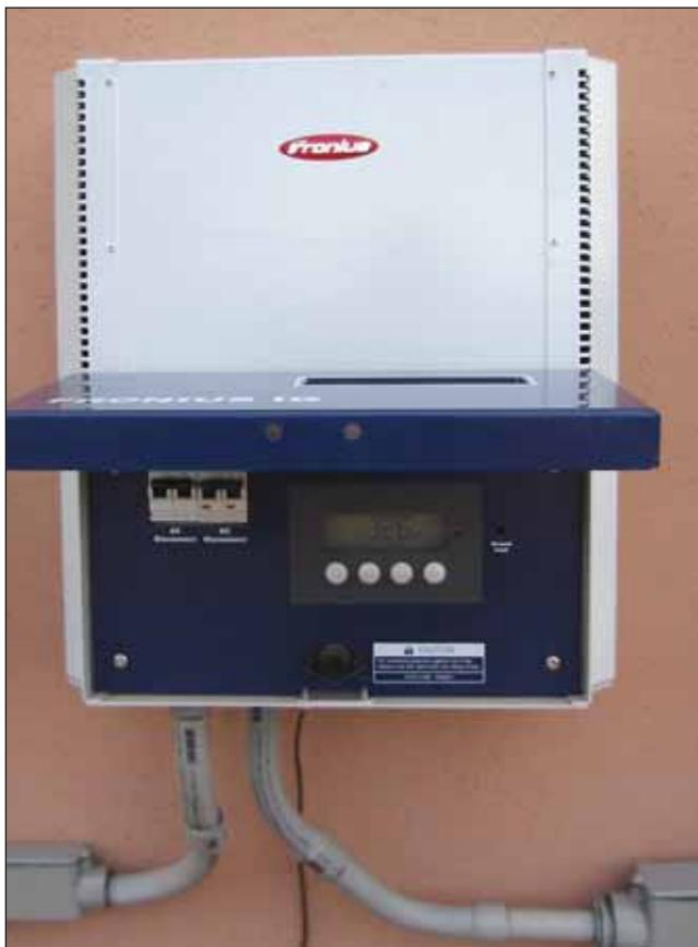
Photo 3. Inverter with internal ac and dc disconnects
