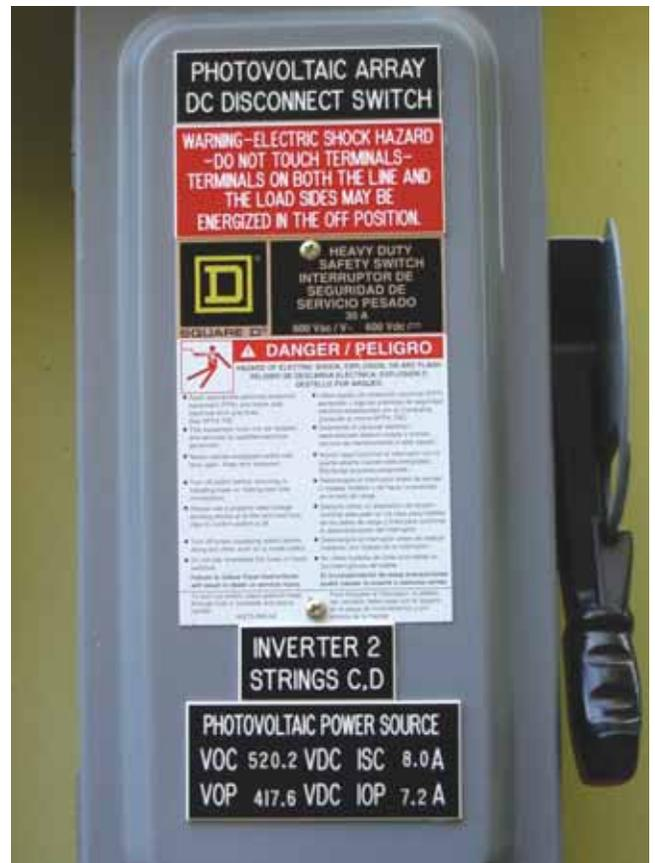
Photo 2. DC PV disconnect with required markings
