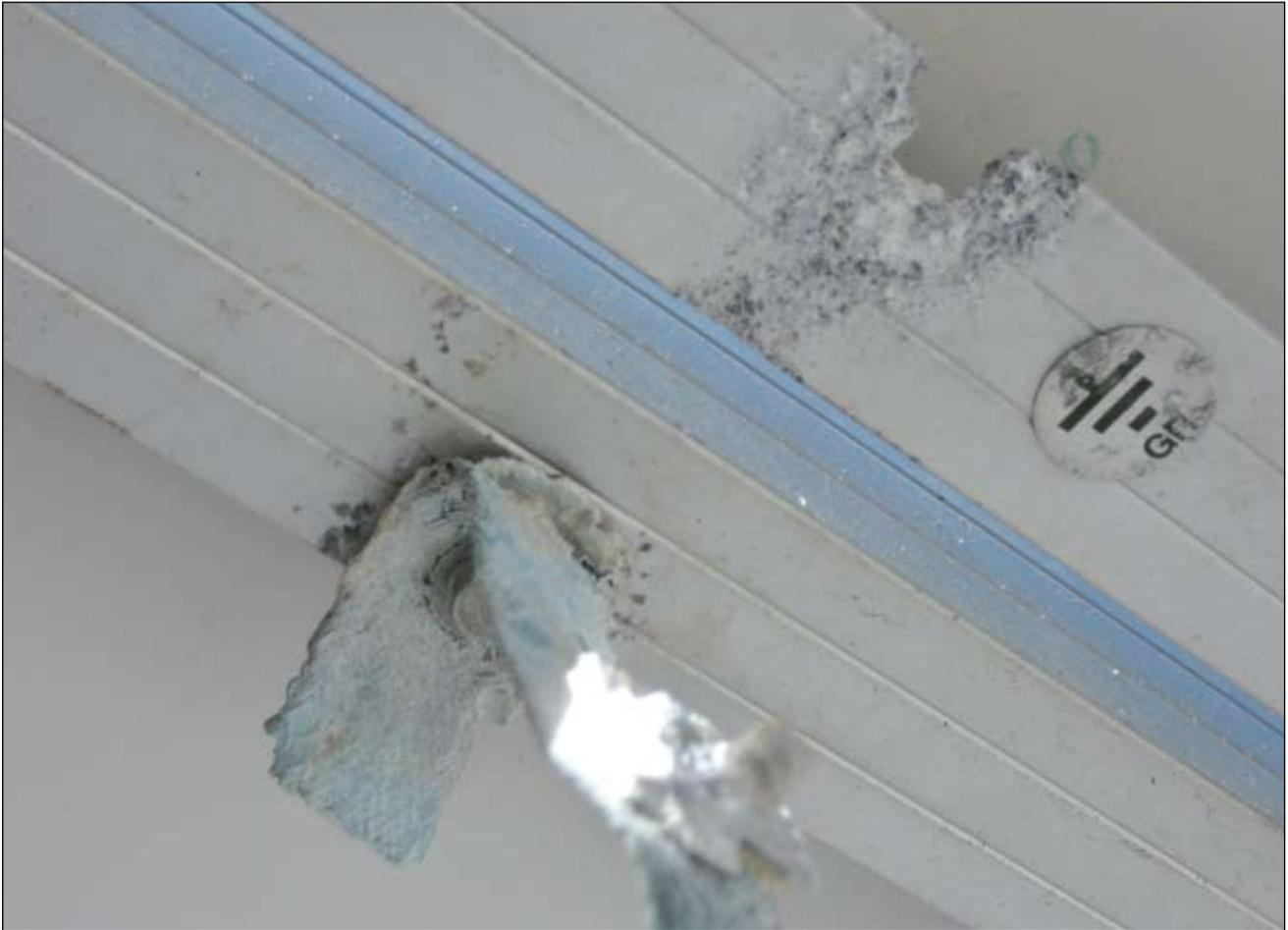
**Photo 2a. Improper module grounding—dissimilar metals**
