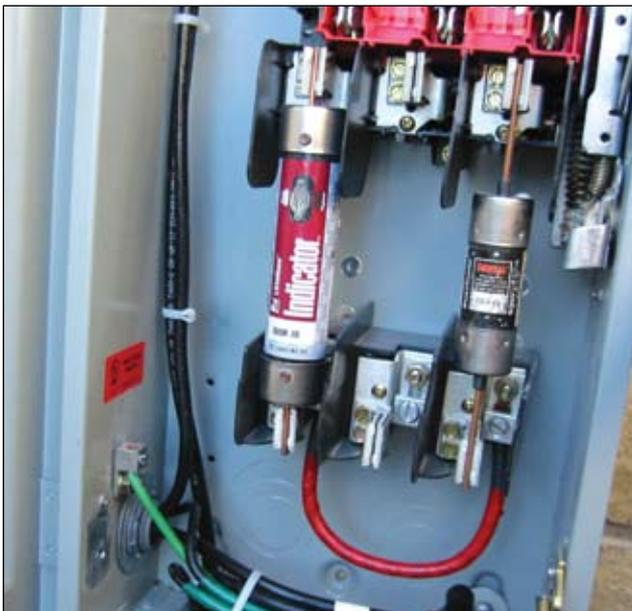
**Photo 4. Improper grounding of enclosure; wrong device, wrong location**
