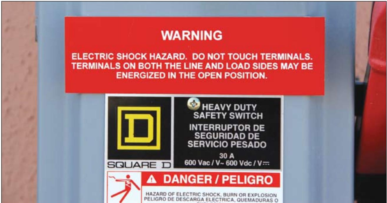
Photo 7. Warning label for PV dc disconnect
