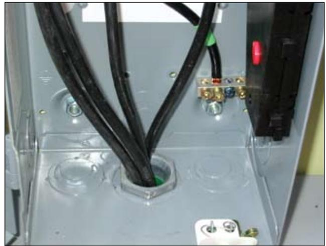
**Photo 5. Listed ground-bar kit in the proper location**
