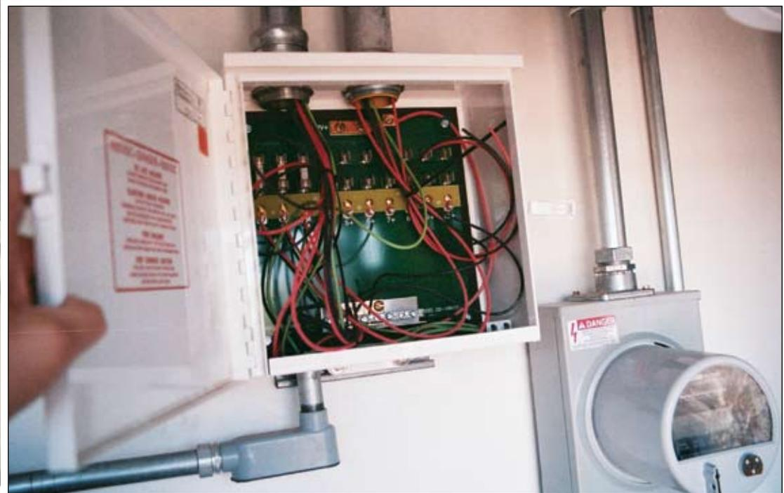
Photo 1. Grounded PV source circuits, but no white conductors
