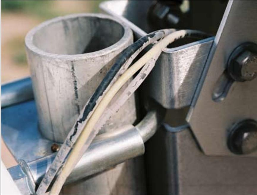
**Photo 8. THHN conductors deteriorating due to outdoor UV exposure**
