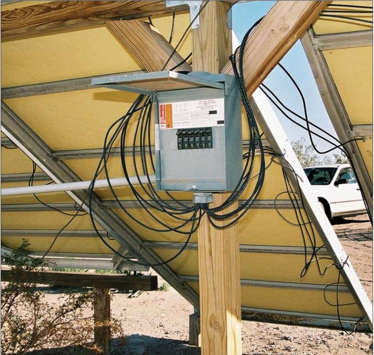
**Photo 2. PV source-circuit combiner with circuit breakers—poor workmanship**
