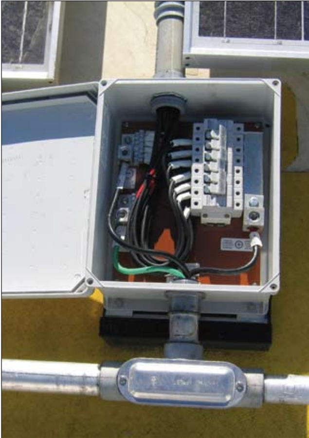
Photo 3. PV source-circuit combiner on large system
