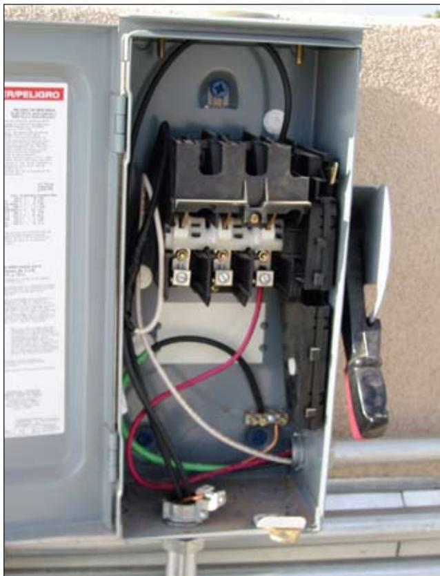
**Photo 7. Line and load connections are important**
