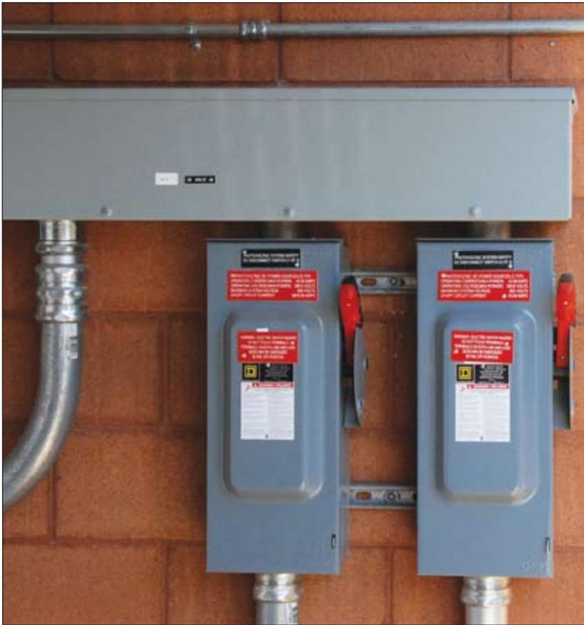
Photo 5. PV dc disconnecting means
