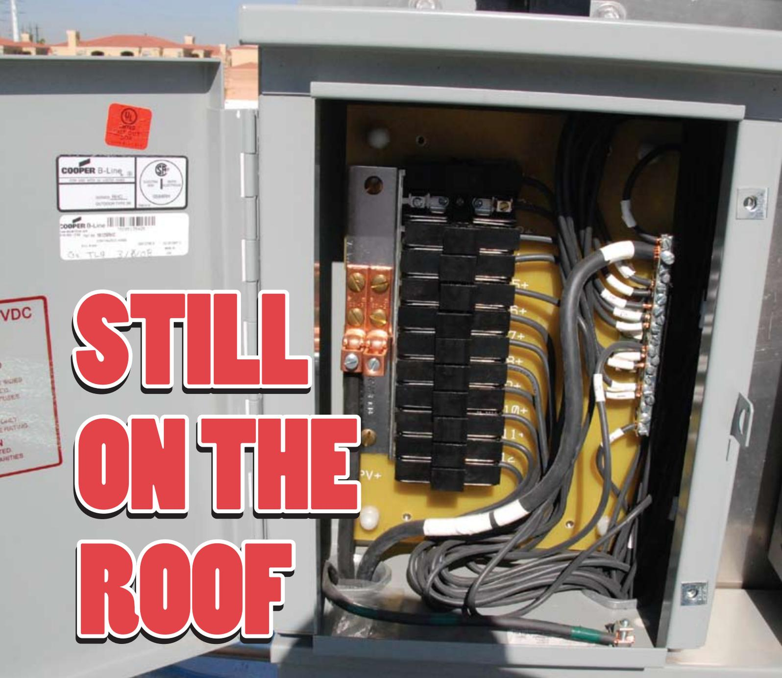
Photo 1. PV source-circuit combiner with fuses
