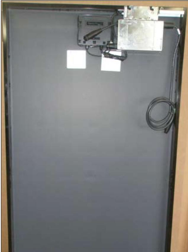
**Photo 4. Almost an AC PV module—just make the dc wiring not accessible**
