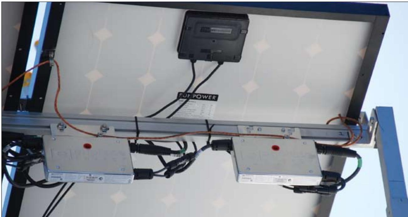
**Photo 2. Pair of Enphase microinverters showing ac and dc cables**
