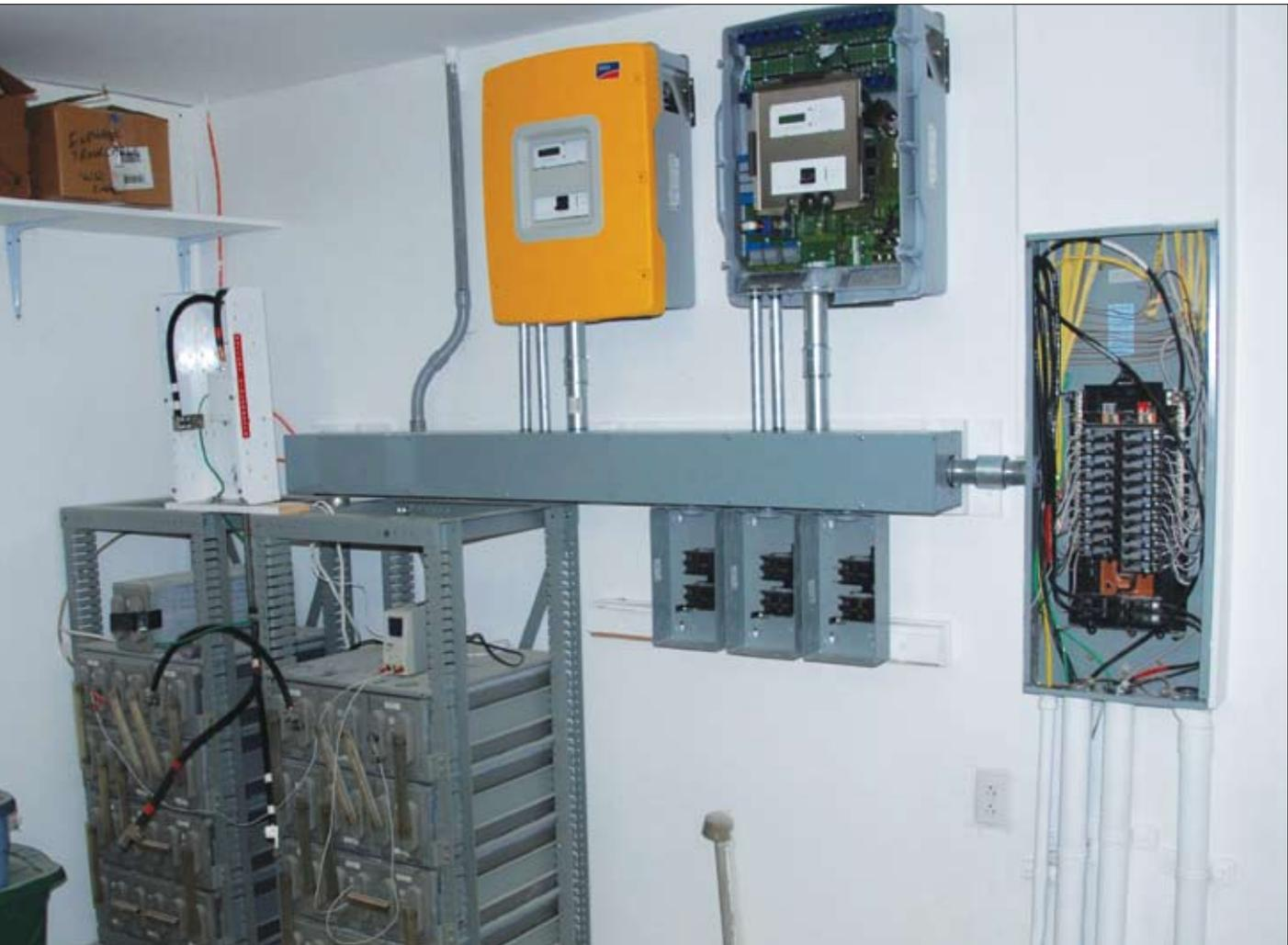
**Photo 1. Battery-backed-up, utility-interactive PV system during installation**
