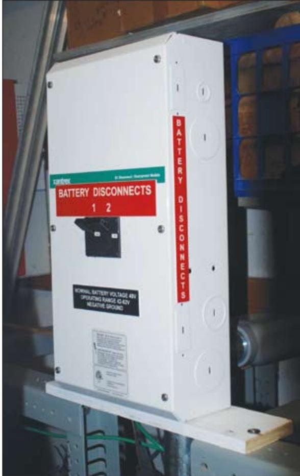
**Photo 4. Battery disconnect and overcurrent protection located near the batteries**
