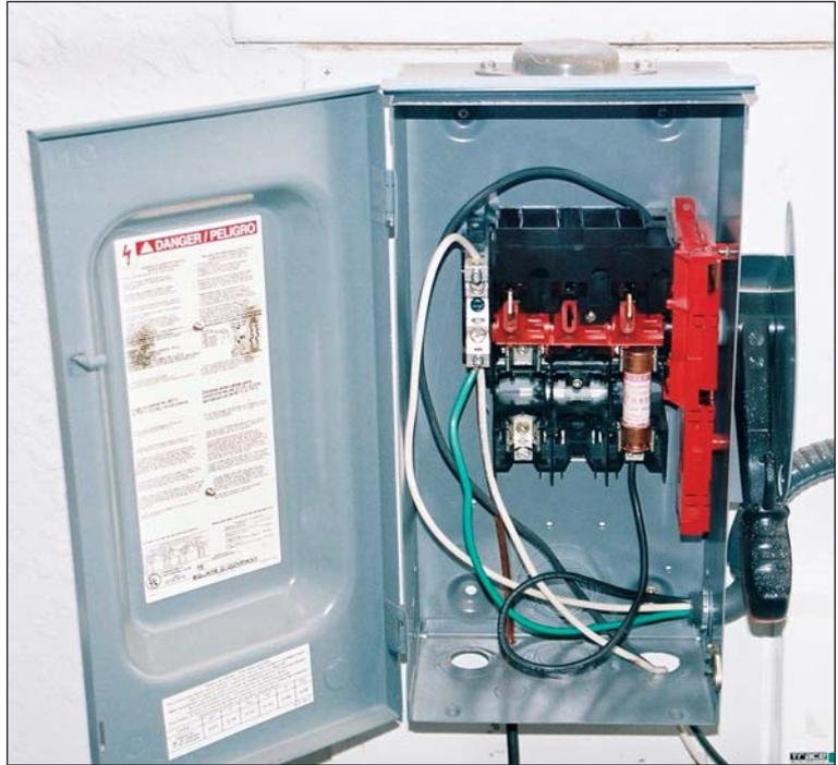
Photo 1. How many conductors can fit in a single terminal?
