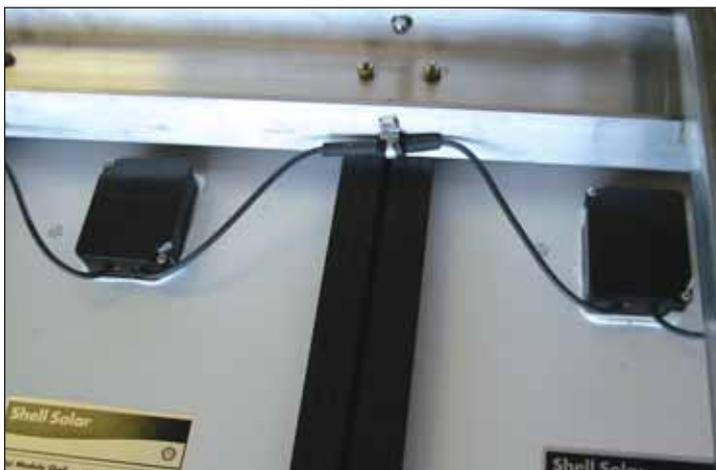
Photo 5. Module wiring properly secured
