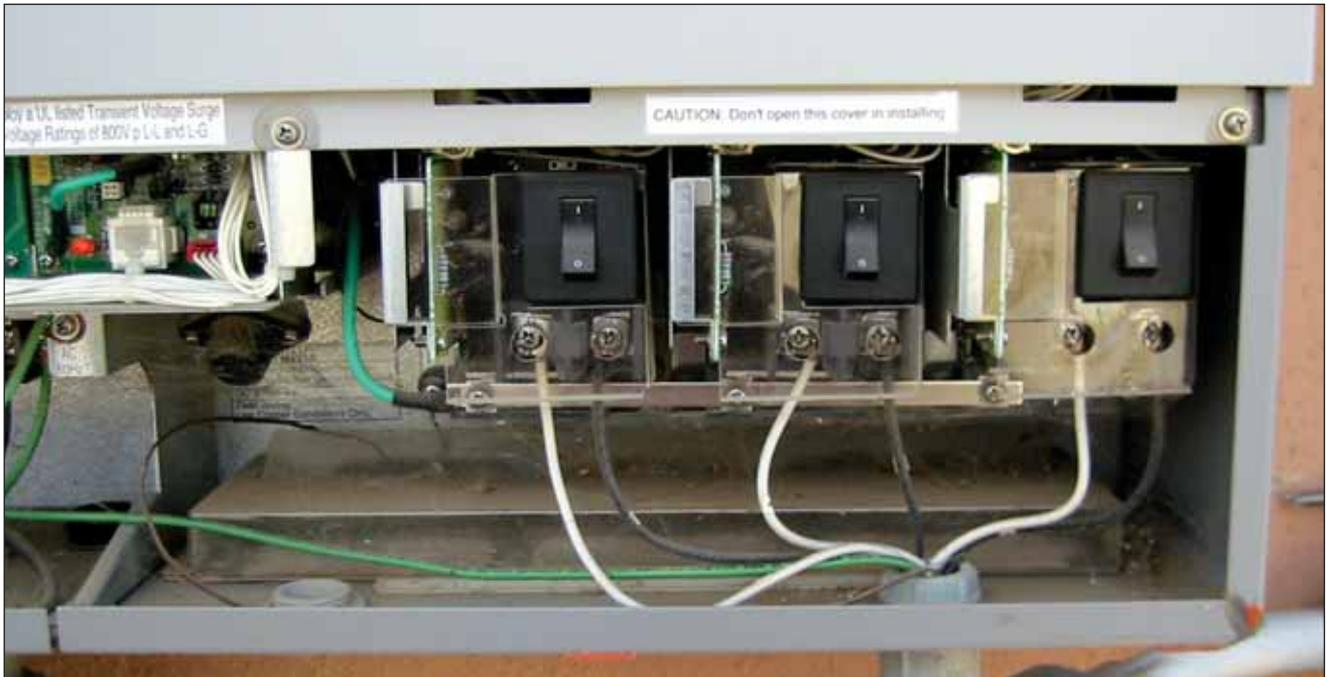
**Photo 2. Inverter with three DC inputs**
