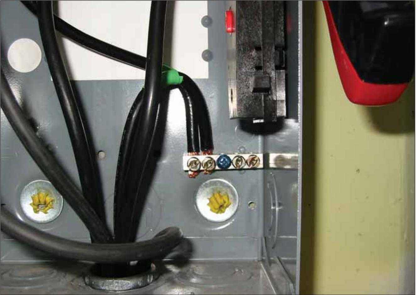
**Photo 4. Properly installed, listed ground bar kit**
