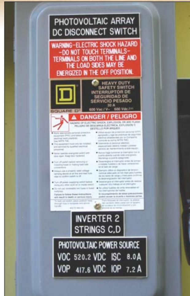
Photo 1. Small system dc PV disconnect
