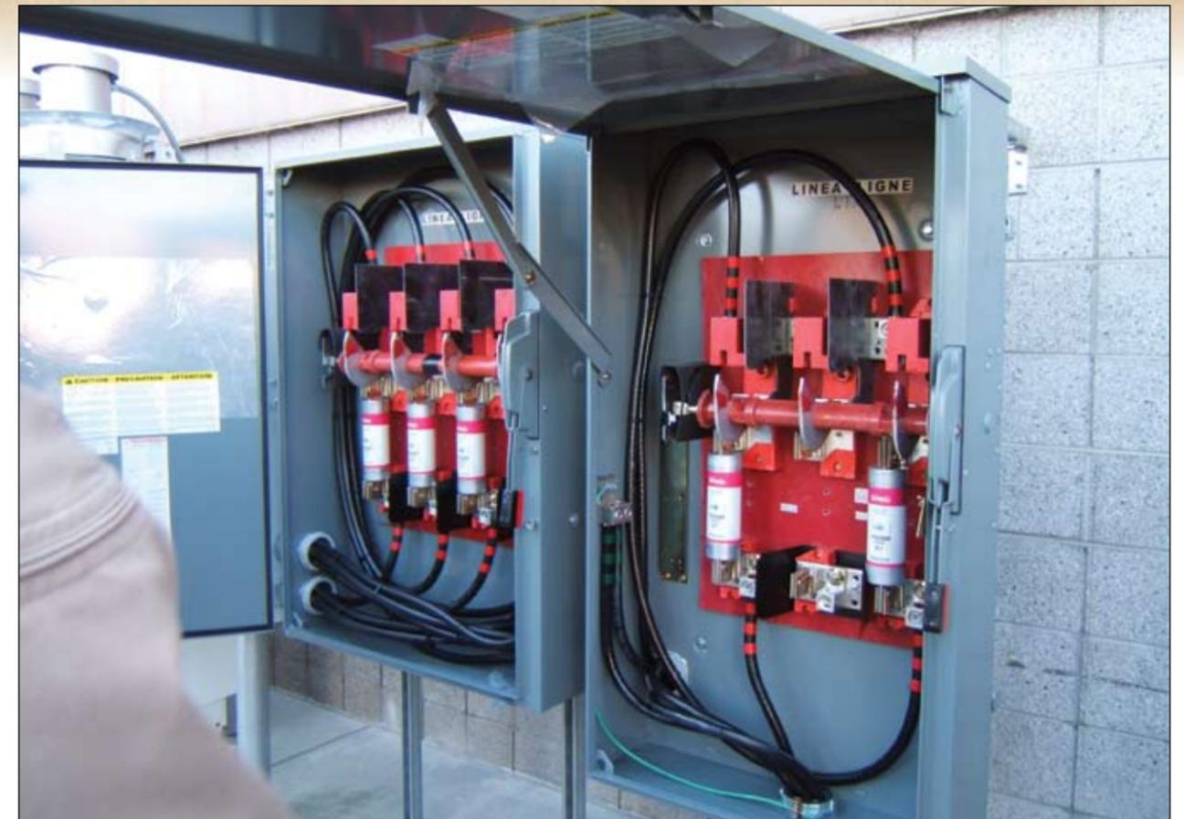
Photo 2. Large system dc PV disconnects
