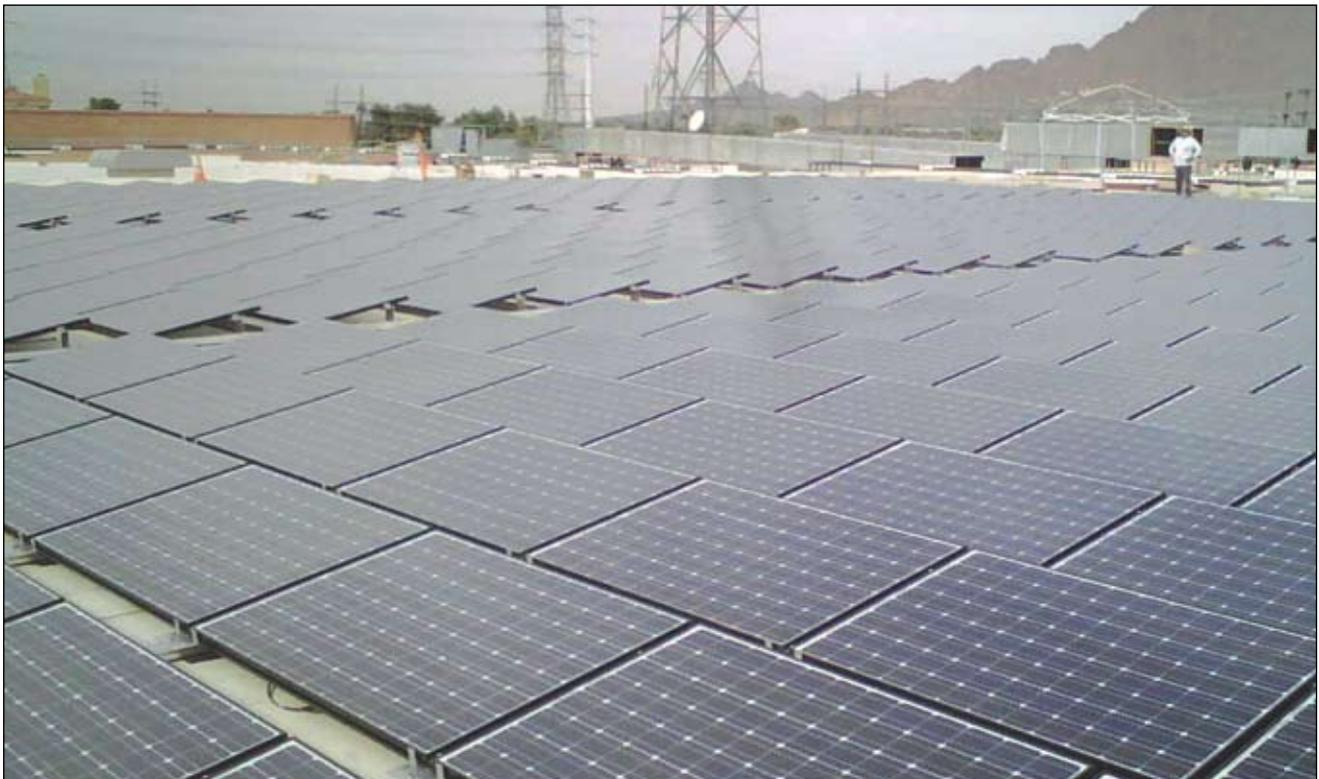
Photo 1a. Large system with multiple strings of modules will require OCPD.
