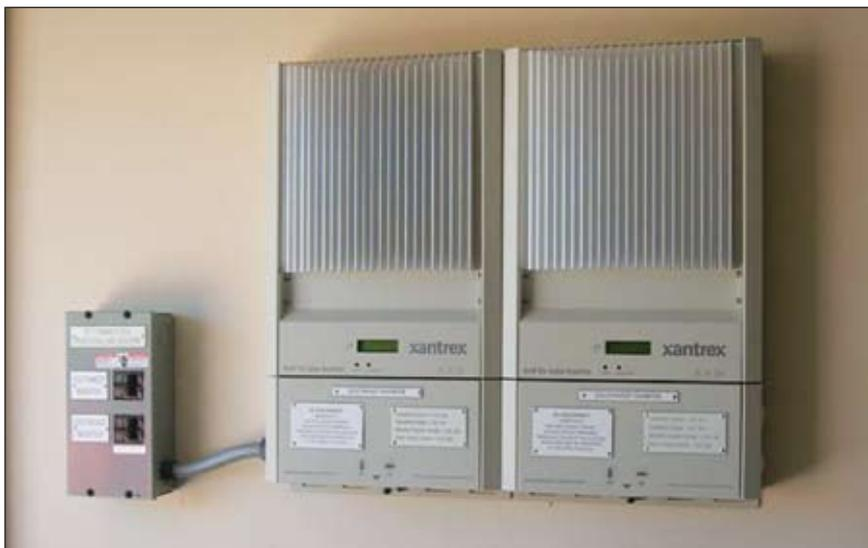
Photo 6. Inverter with internal disconnects that can be separated from inverter
