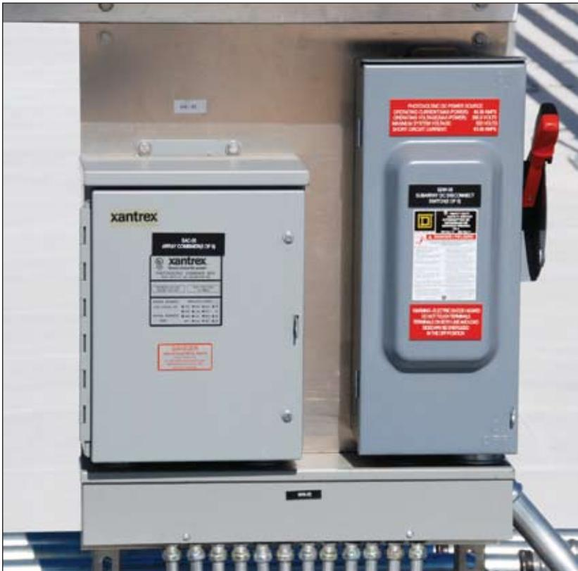
Photo 7. PV combiner with disconnect at output
