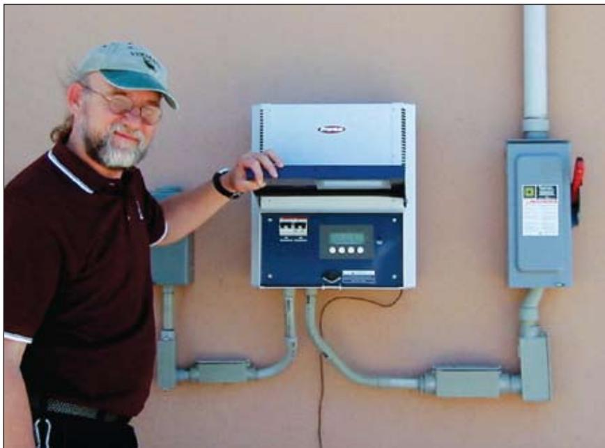
Photo 5. Inverter with internal disconnects as part of the inverter
