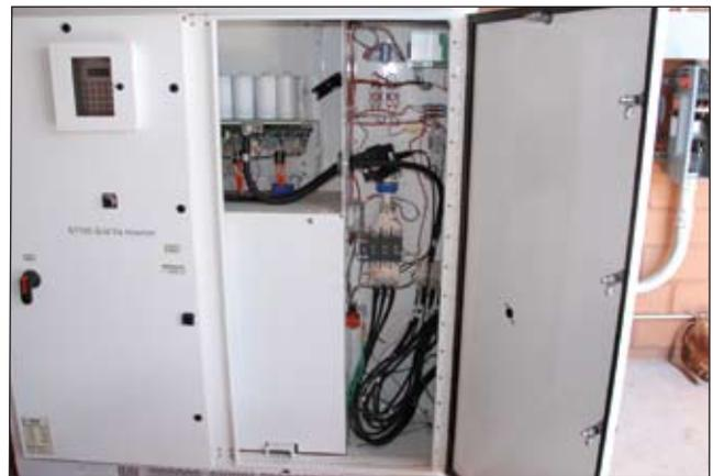
Photo 2. Xantrex 100kW Inverter
