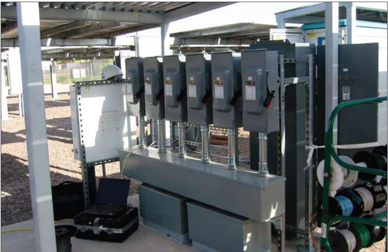
Photo 8. Disconnects for each input installed near the inverter
