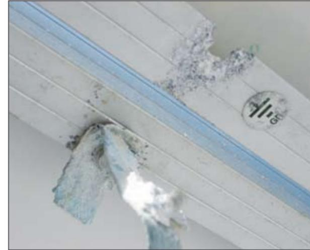
Photo 6. Tinned copper braid offers no protection for aluminum module frame.
