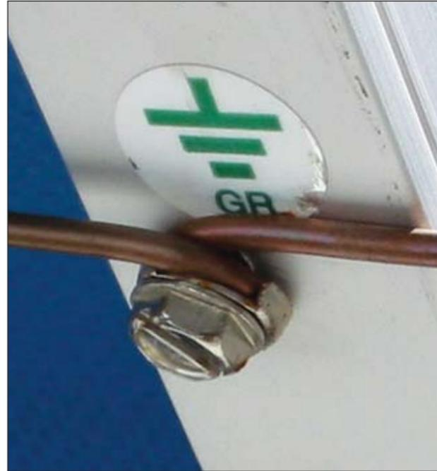
Photo 4. Installed per instruction manual—but copper touching aluminum?
