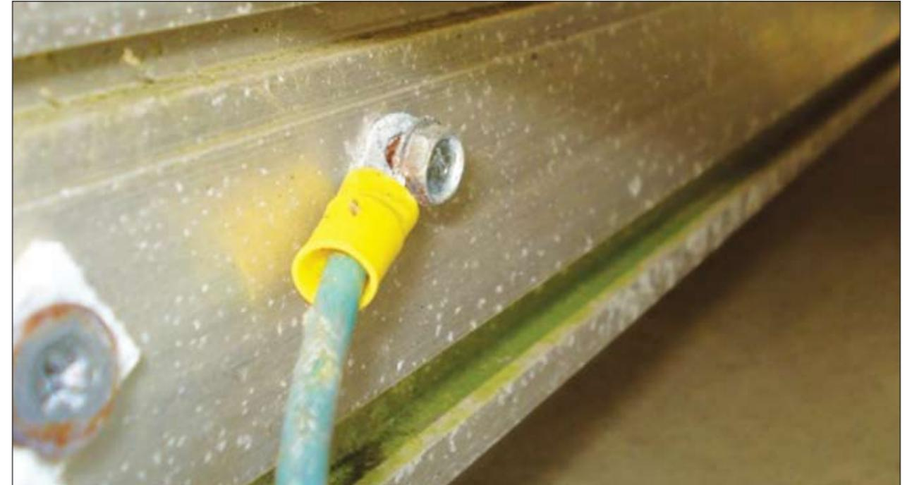
Photo 2. Improper lugs and conductors. Not securely fastened.
