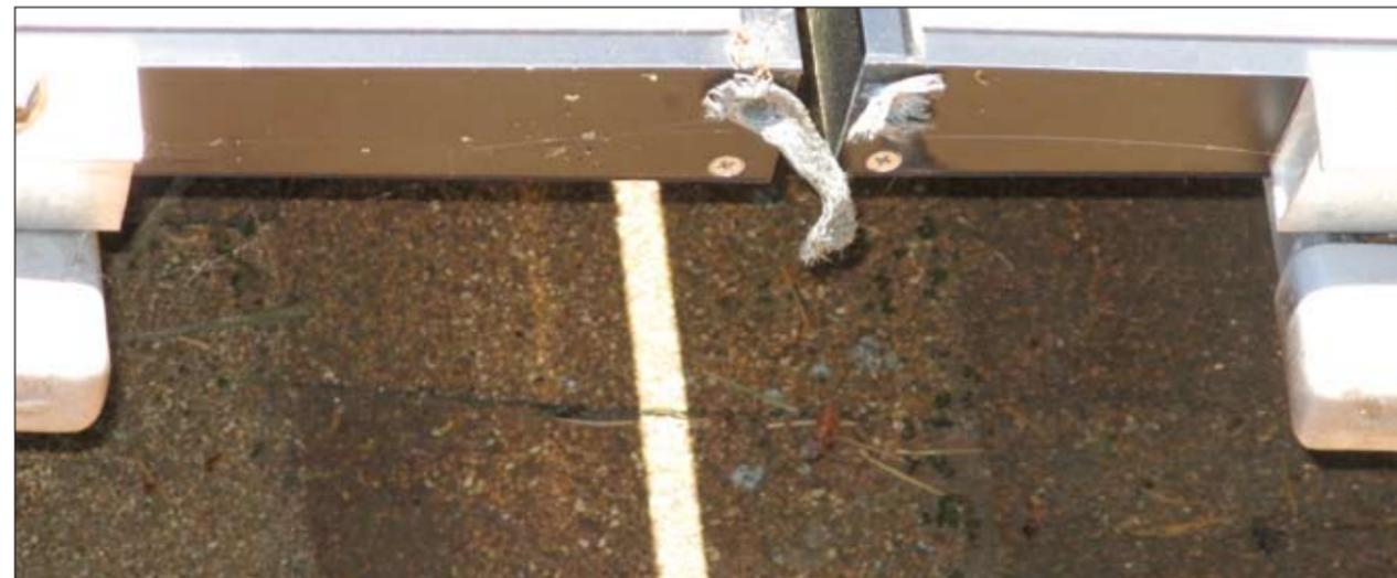
Photo 5. Improper use of module bonding screw and copper in braid touching aluminum.
