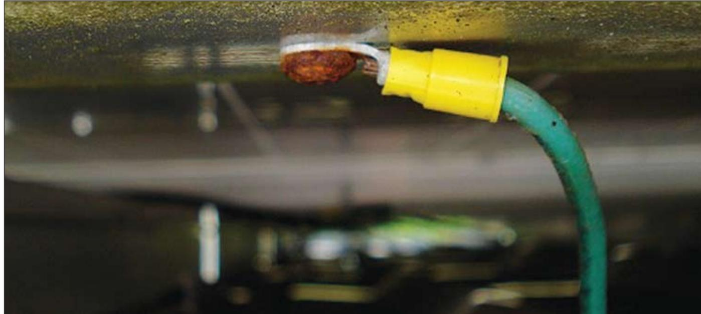
Photo 1. Improper module grounding: Plated steel thread cutting screw is not corrosion resistant; THHN conductors and nylon lug are not UV-rated.
