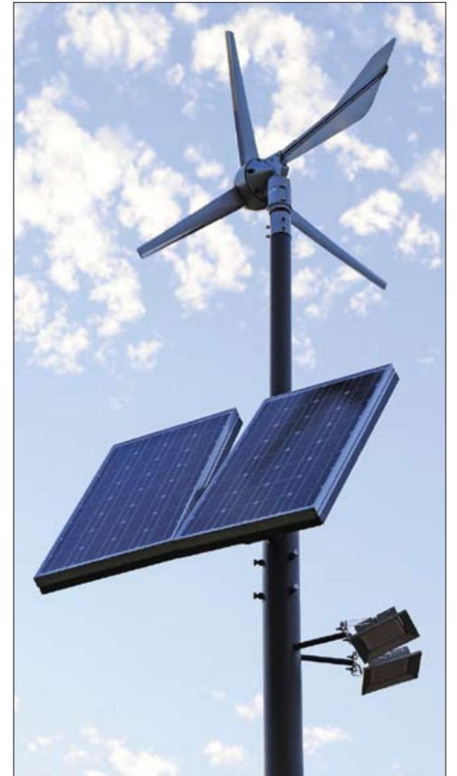
Photo 4: Small wind system combined with solar panels
