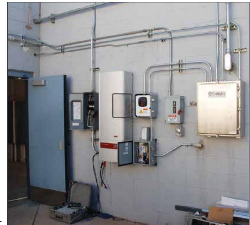
**Photo 4. Oops, ac disconnect on other side of the wall**
