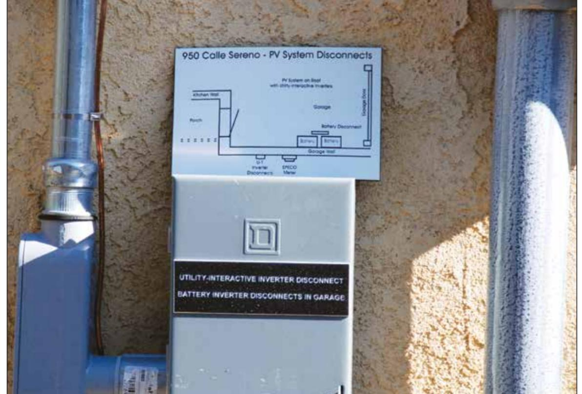
**Photo 2. Placard showing external ac PV disconnect and dc battery disconnect in garage.**
