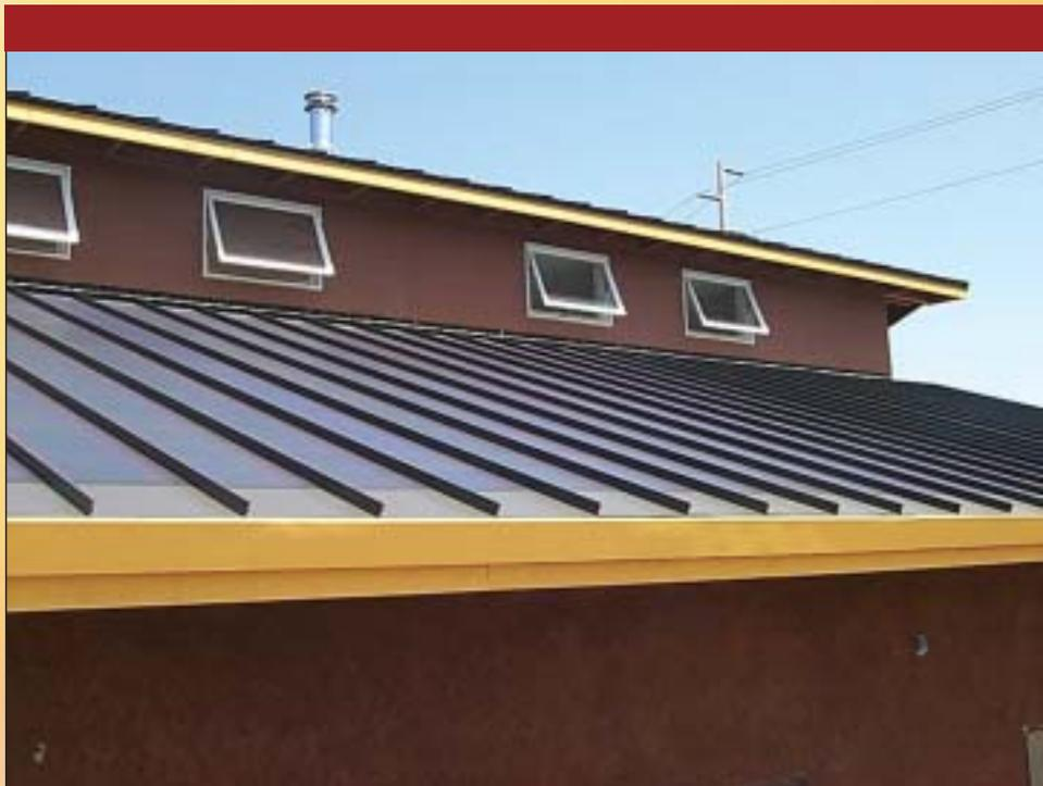
Photo 3. PV modules laminated to metal roof
