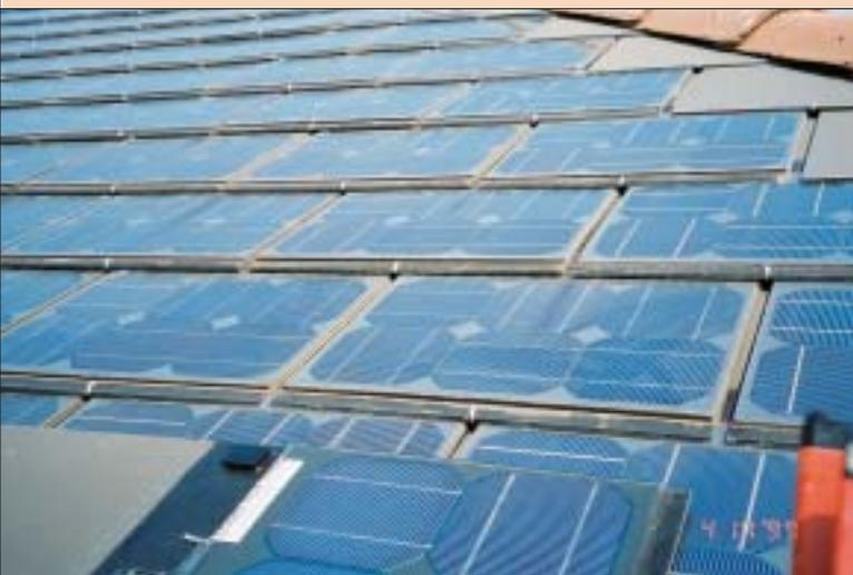
Photo 2. PV modules as roofing material
