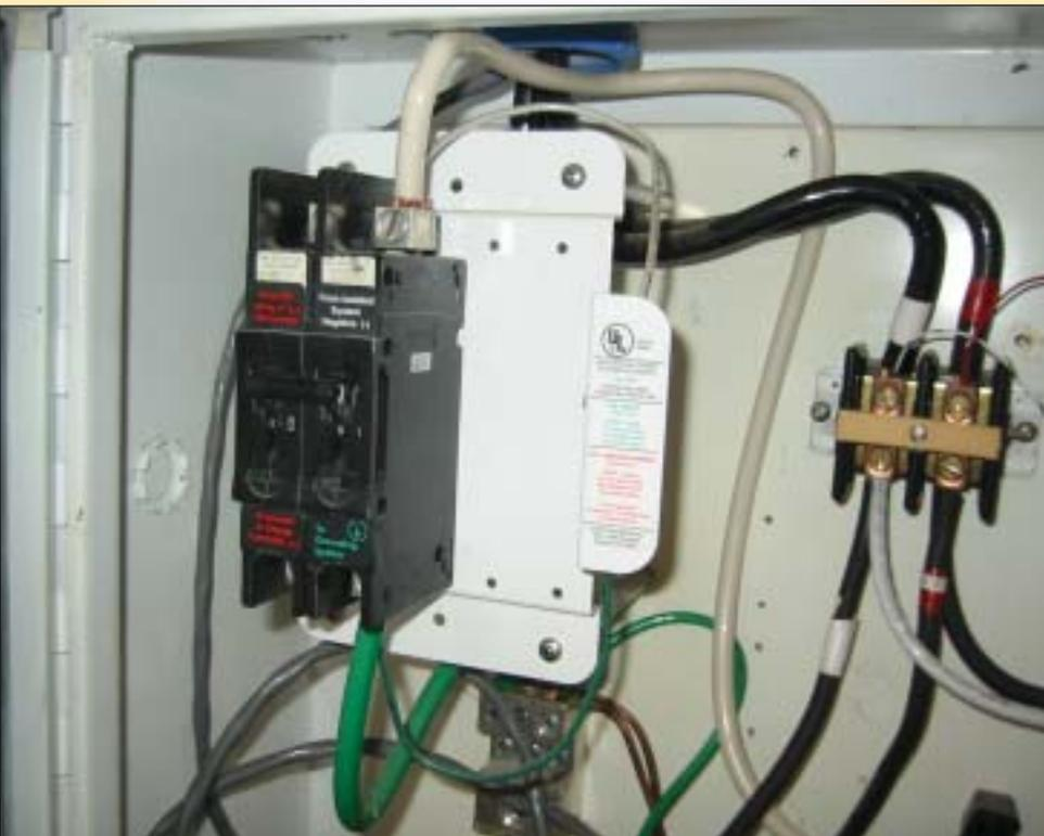
Photo 12. Stand-alone PV ground-fault protection device
