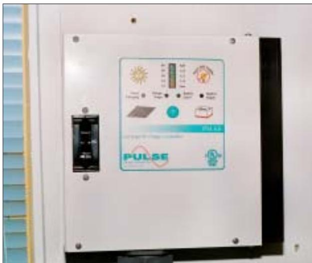
Photo 7. 60 A PV charge controller
