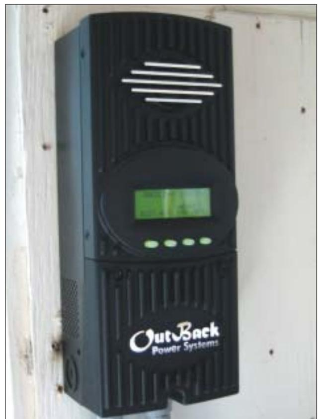
Photo 8. 60 A max power tracking PV charge controller
