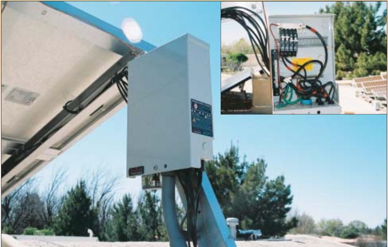
Photos 5 and 5A. PV combiner with circuit breakers
