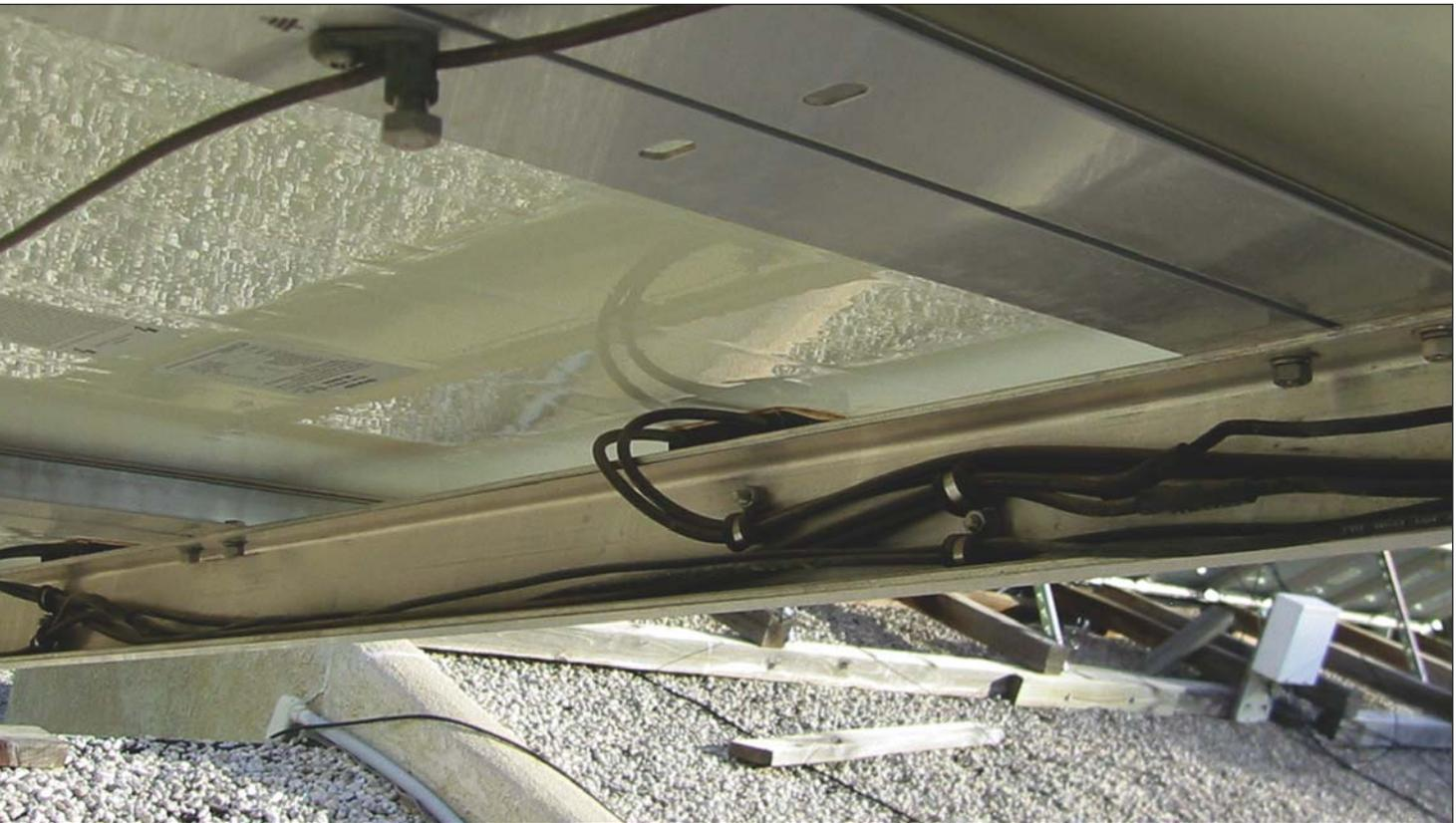
**Photo 2. Pipe clamps with inserts holding cables securely**
