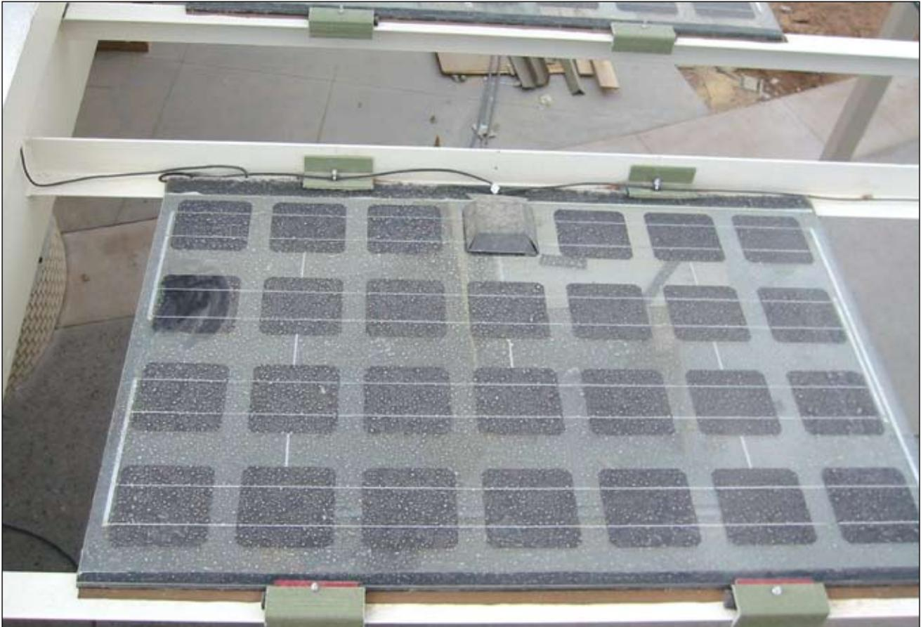
**Photo 3. Frameless PV modules in overhead canopy**
