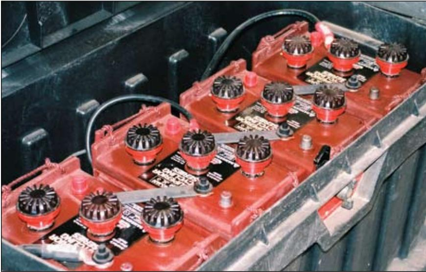
**Photo 7. Flooded, lead-acid batteries in containers**
