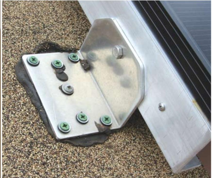
**Photo 2. Module rack mounting bracket**
