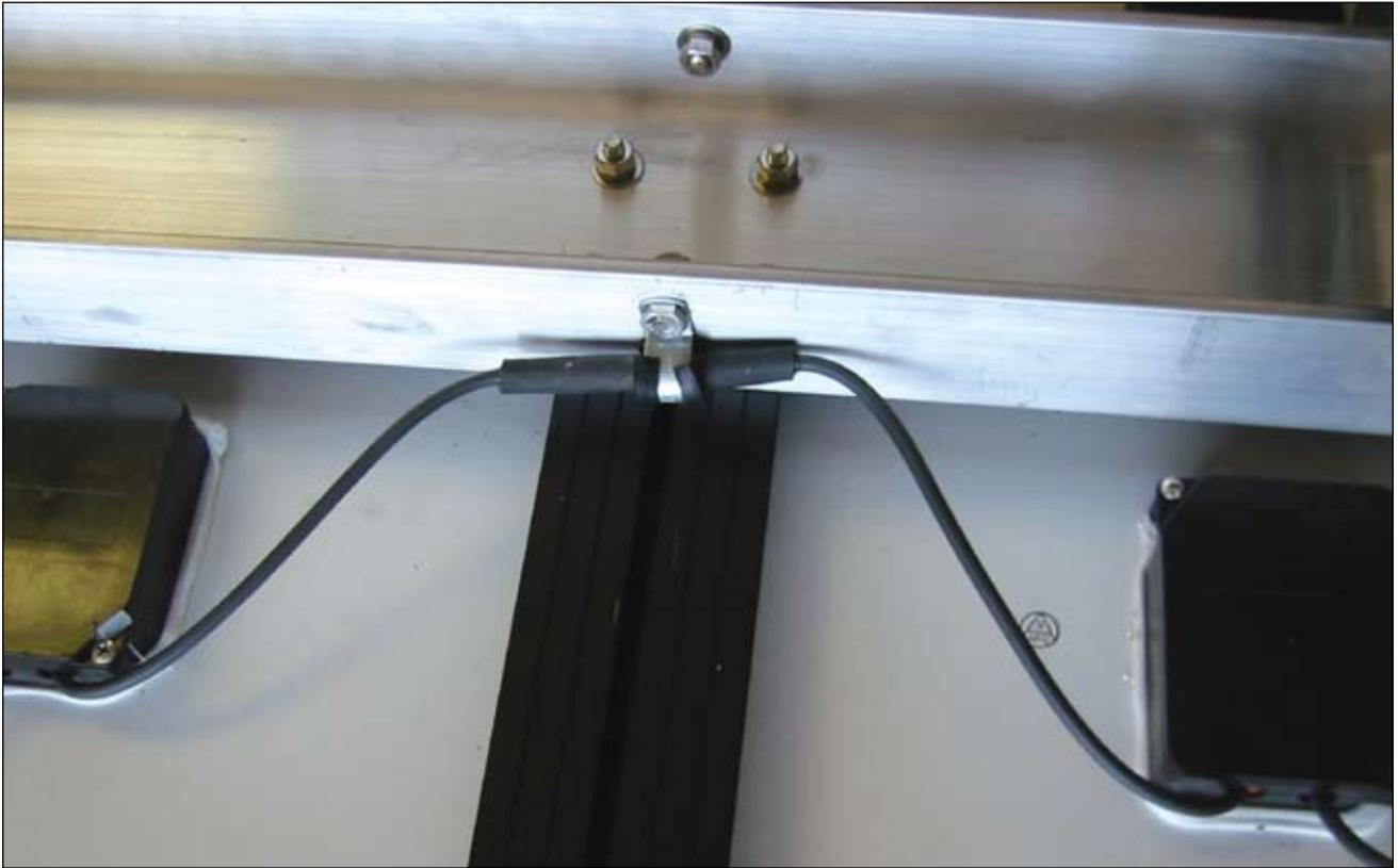
**Photo 5. Shortened, spliced, and secured module interconnections**
