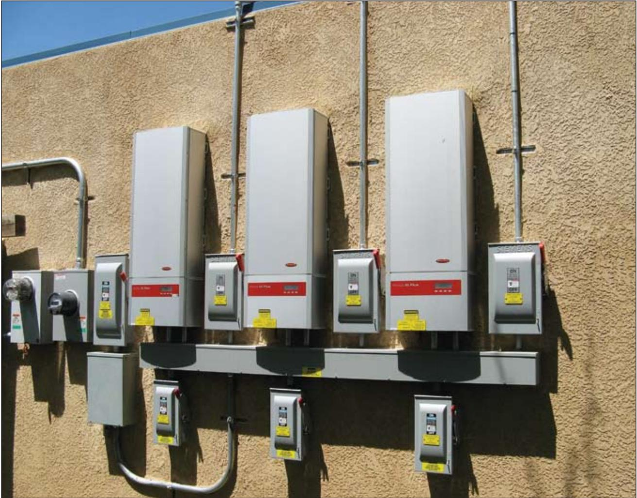
**Photo 2. Multiple inverters require special connections**
