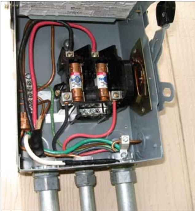
Photo 4. Utility-required disconnect, fused
