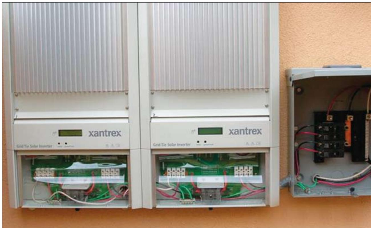
**Photo 3. Two inverters with PV ac combining panel**
