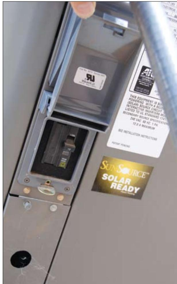
Photo 9. Backfed PV breaker in power panel on outdoor unit
