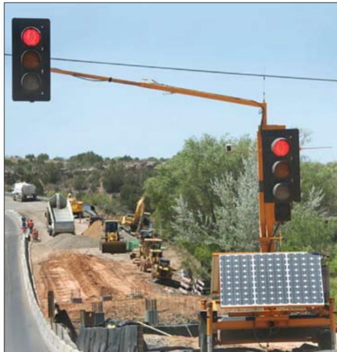
Photo 4. PV-powered construction sign.
