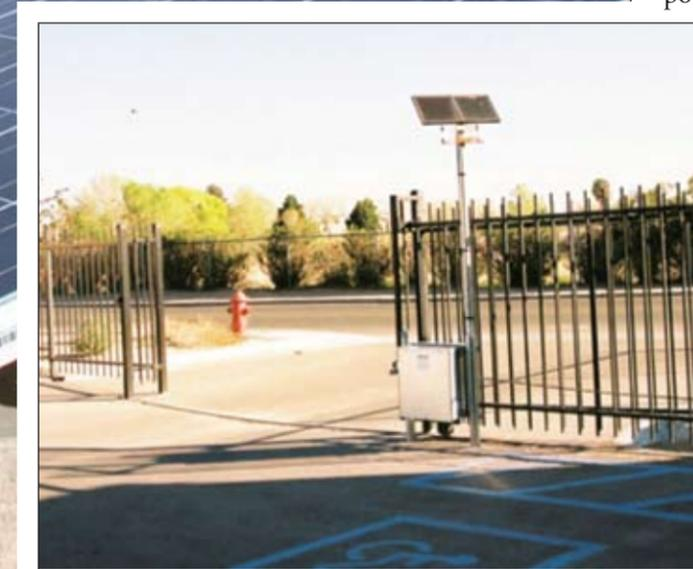
Photo 1. PV-powered electric gate; no trenching required
