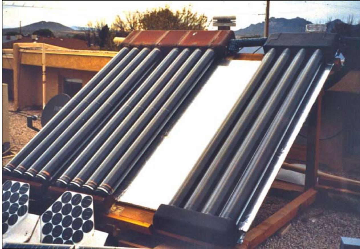
Photo 3. Solar water collector and PV modules connected to the circulating pump
