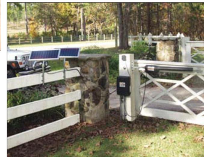
Photo 2. PV-powered electric gate. Courtesy MightyMule/GTO
