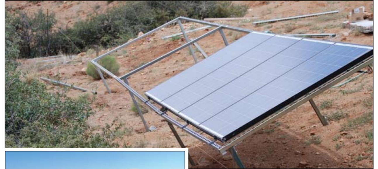
Photo 10. Four AC PV modules installed with expansion room for more modules
