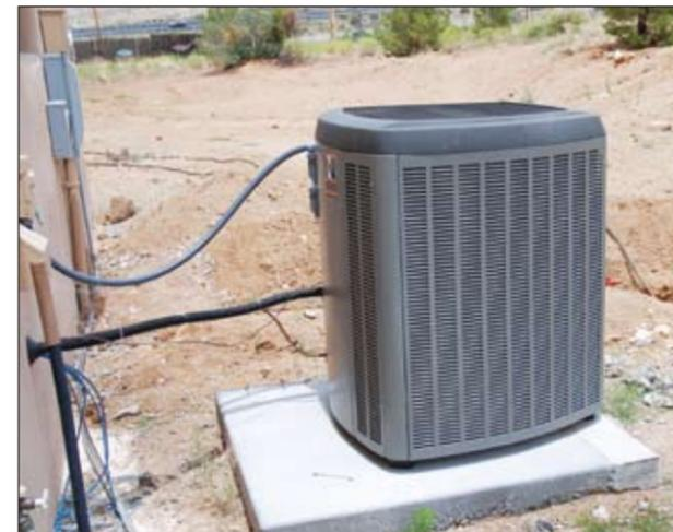
Photo 6. Lennox XC-21 SunSource Air Conditioning Outdoor Unit connections to make and inspections are usually not justifiable.
