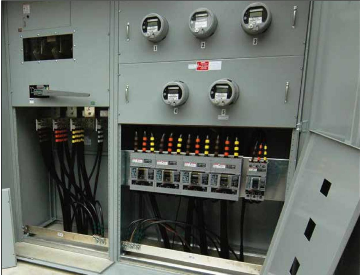
**Photo 4. Large system electrical switchgear. Possible connection points must be identified and made by an approved organization and allowed by the utility.**
