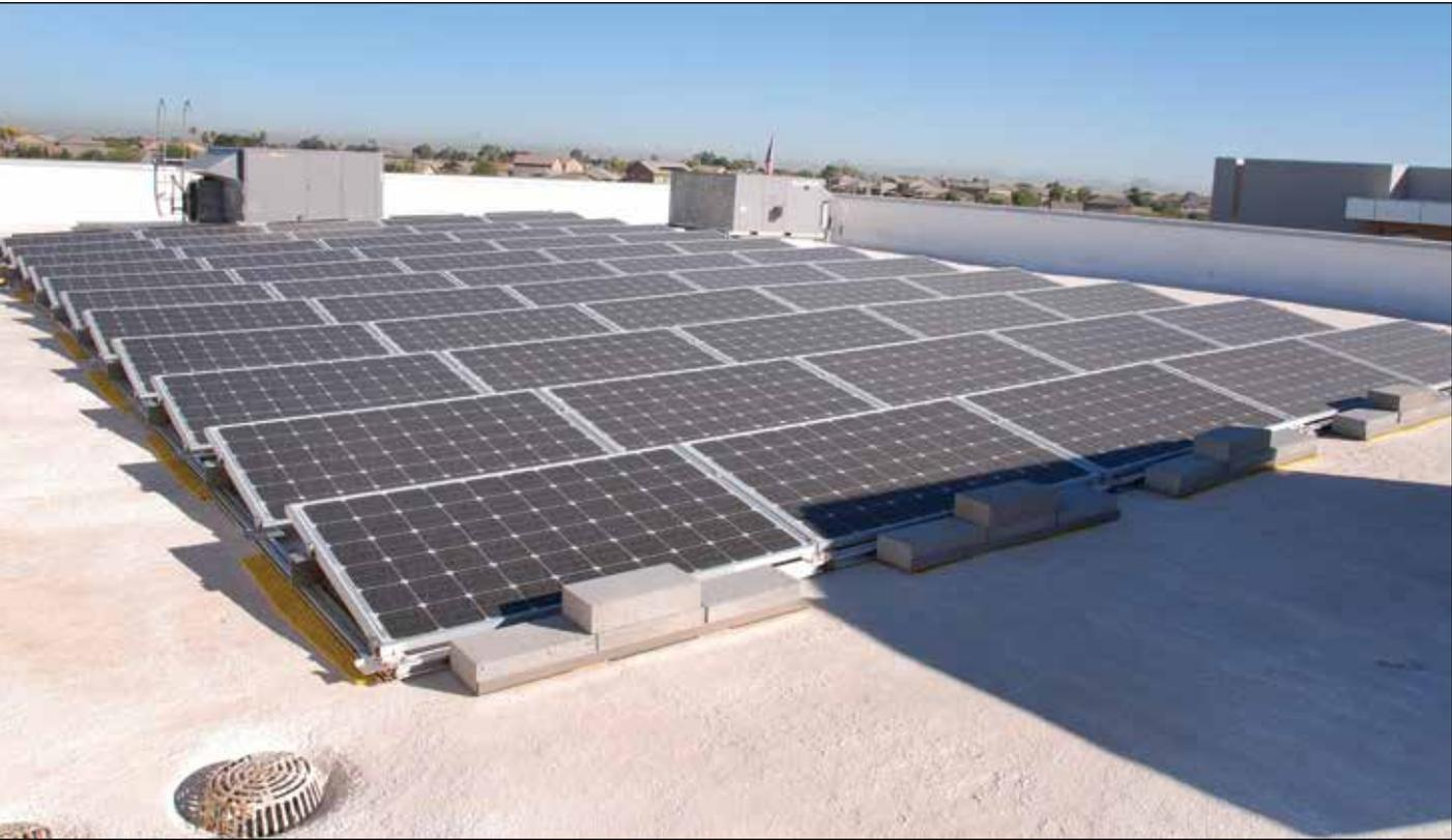
**Photo 1. PV systems are getting larger and frequently will require supply-side connection to the utility. No, shaded modules are not good and will not get the maximum energy from the PV array.**
