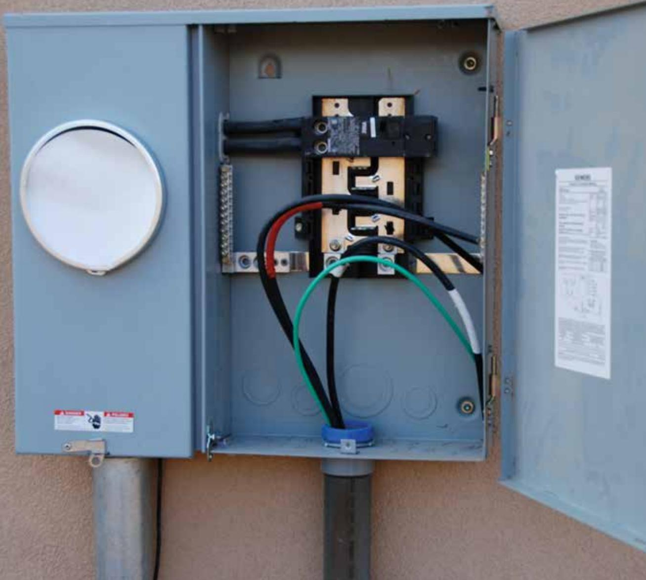
**Photo 3. Meter main combos may not have the internal conductors (or bus bars) tapped for a PV supply-side connection. Such a connection would violate the listing on the device and therefore violate NEC section 110.3(B).**
