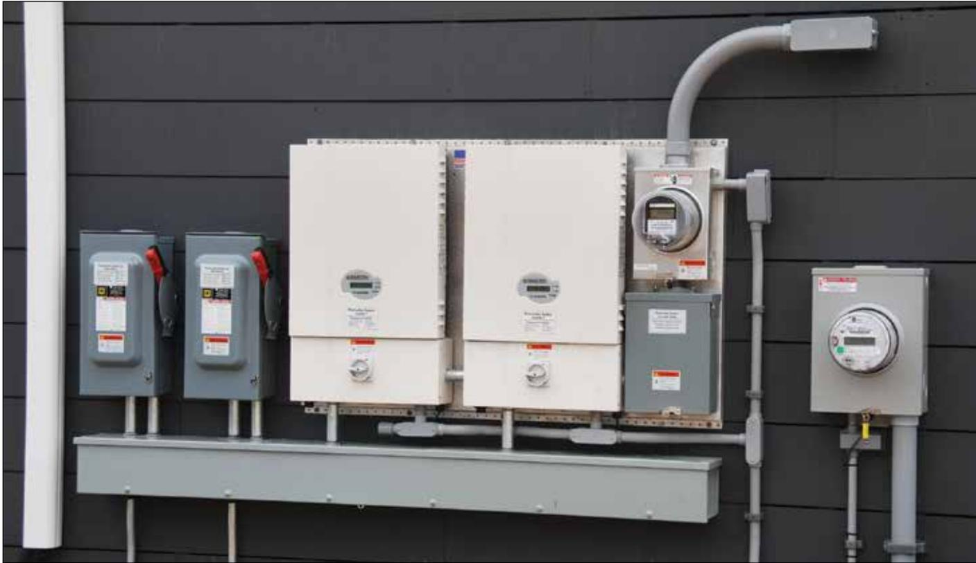
**Photo 2. Two inverters on a residential installation will generally indicate that a supply-side utility connection is required.**
