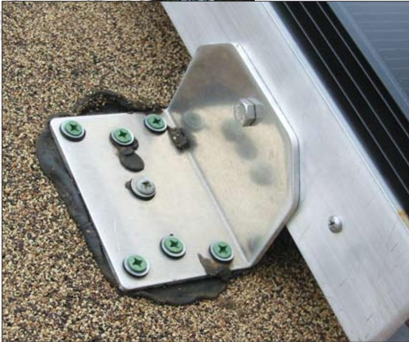
**Photo 1. Array rack attachment point—used in dry climates**
