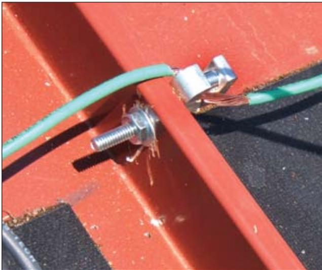
Photo 6. Grounding a metal roof—Oops, outdoor rated lug and wire needed
