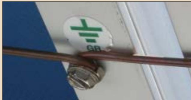
Photo 5. Improperly installed grounding hardware
