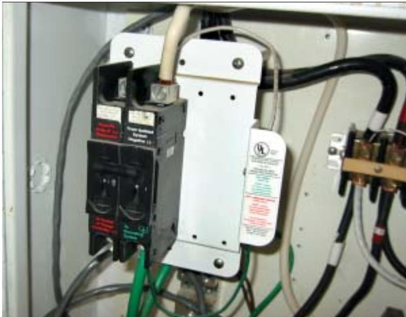
Photo 6. External ground-fault protection device
