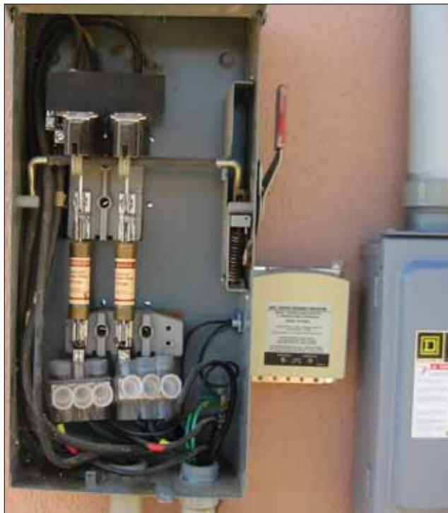
**Figure 3. PV inverter output connected to service conductors**
