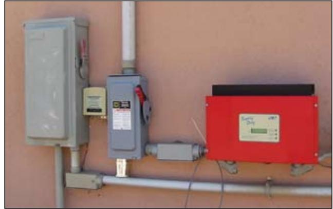
**Photo 1. DC PV disconnect grouped with ac service disconnect**
