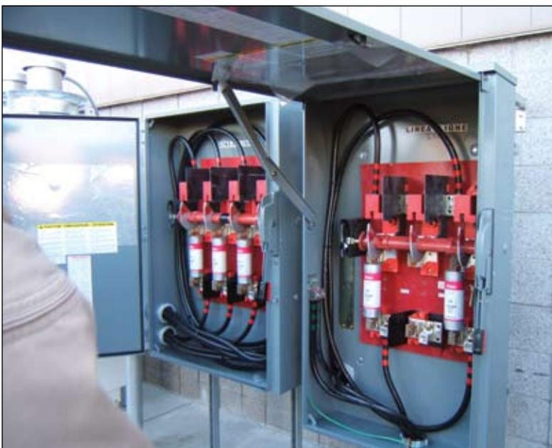
**Photo 2. High-current dc fusing**
