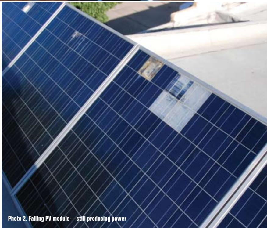
Photo 2. Failing PV module—still producing power
