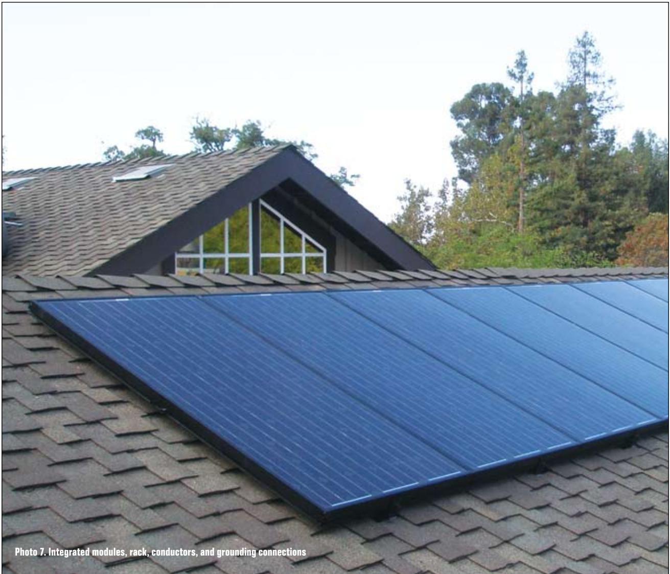
Photo 7. Integrated modules, rack, conductors, and grounding connections
