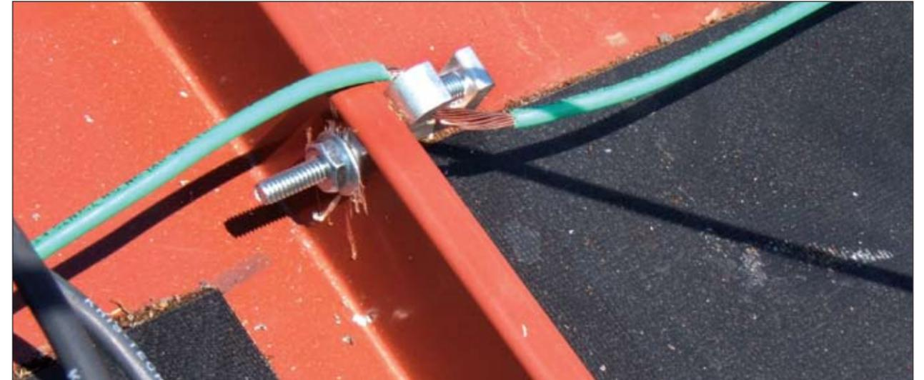
Photo 4. Incorrect conductor being used outdoors
