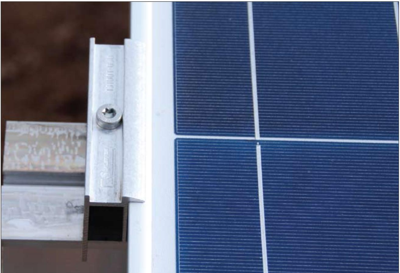
Photo 1. Top of frame module mounting. Listing is valid only if the method is in the instruction manual.
