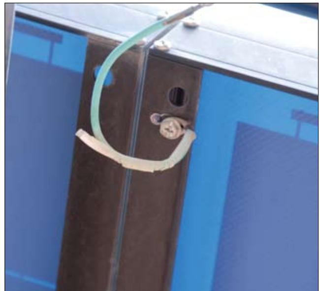
Photo 5. Right grounding point; wrong hardware and method.
