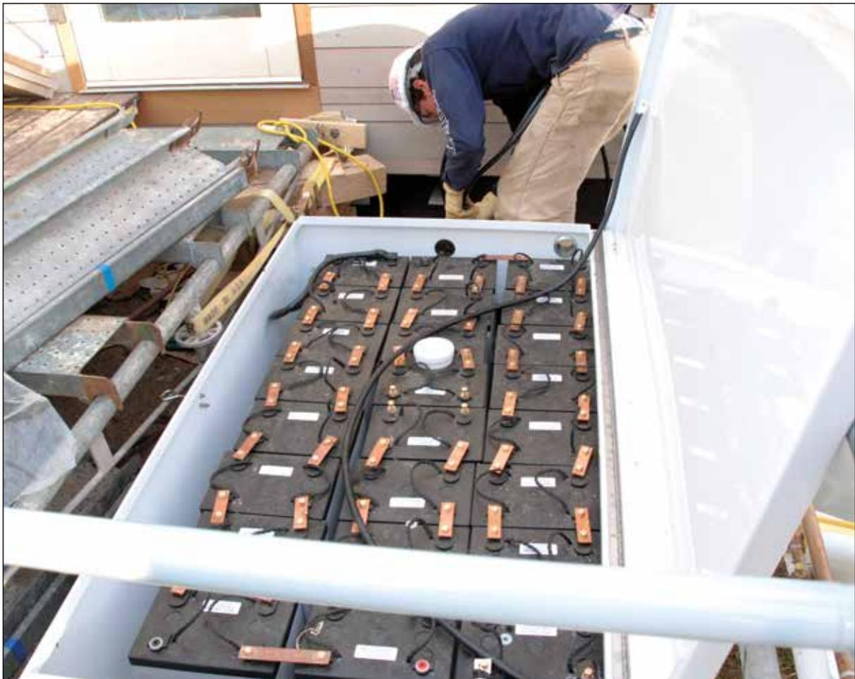
**Photo 2. Valve Regulated Lead Acid (VRLA) batteries**
