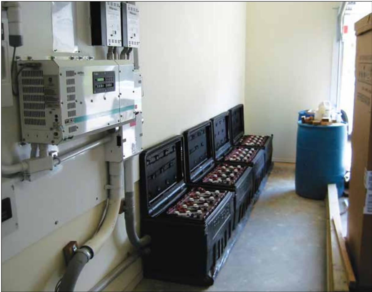
**Photo 3. Flooded lead acid batteries in polyethylene containers**
